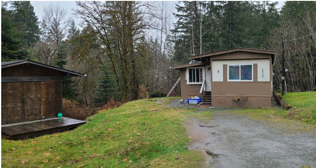
West half of the property viewed from Plested Road, showing the mobile home and detached accessory structure.
