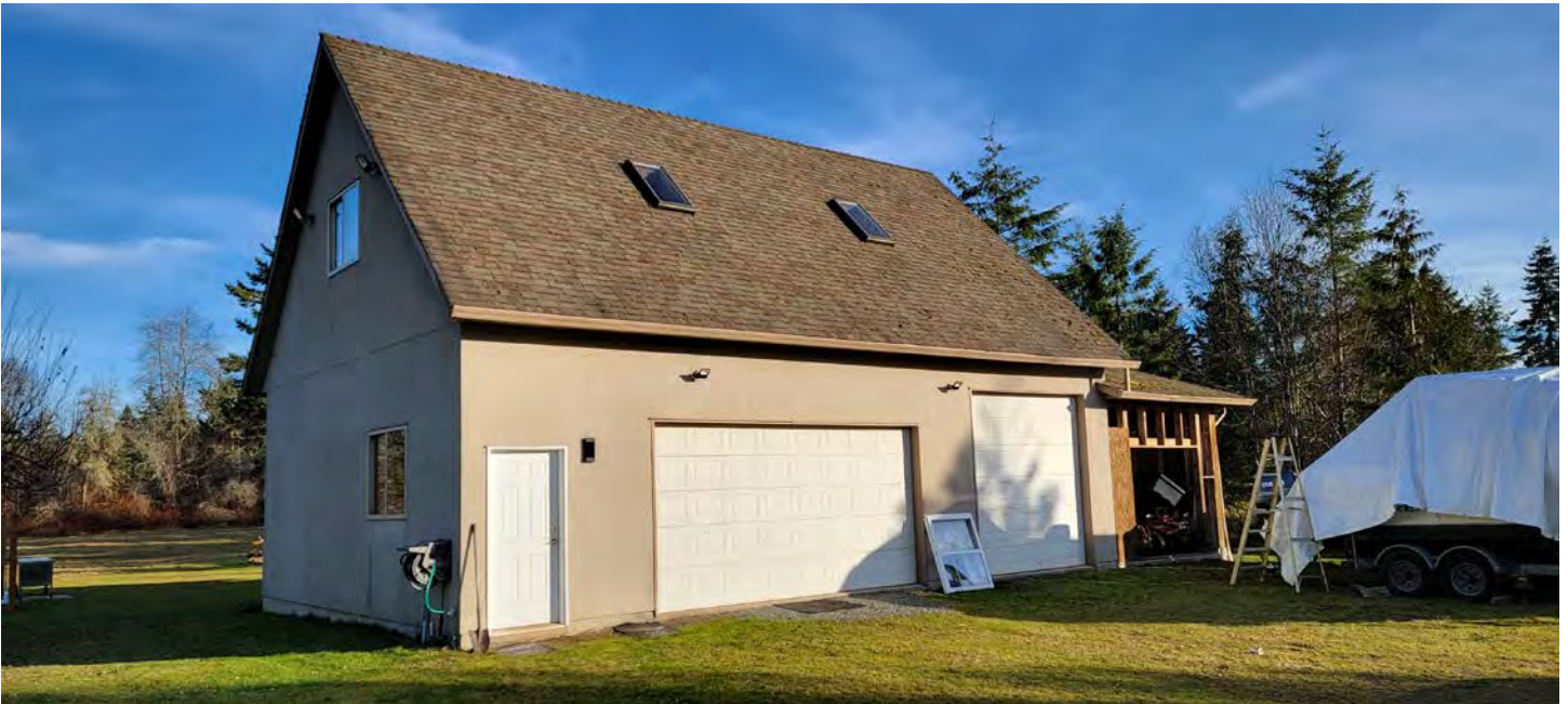
Detached garage structure on property.
