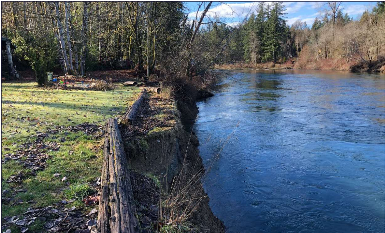
Figure 2.6.1 – Typical Foreshore Conditions (View Looking South)
