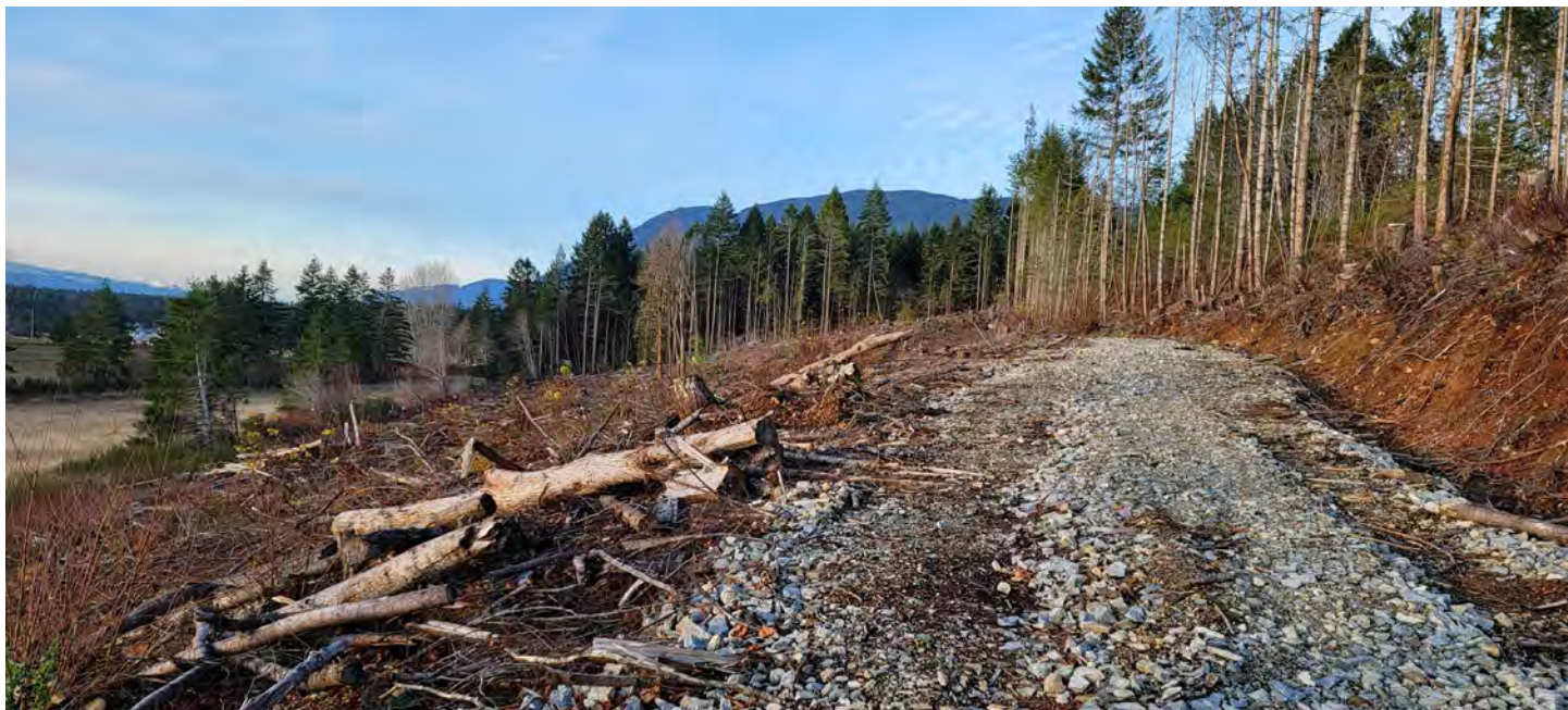
Looking north along internal access road on the property.
