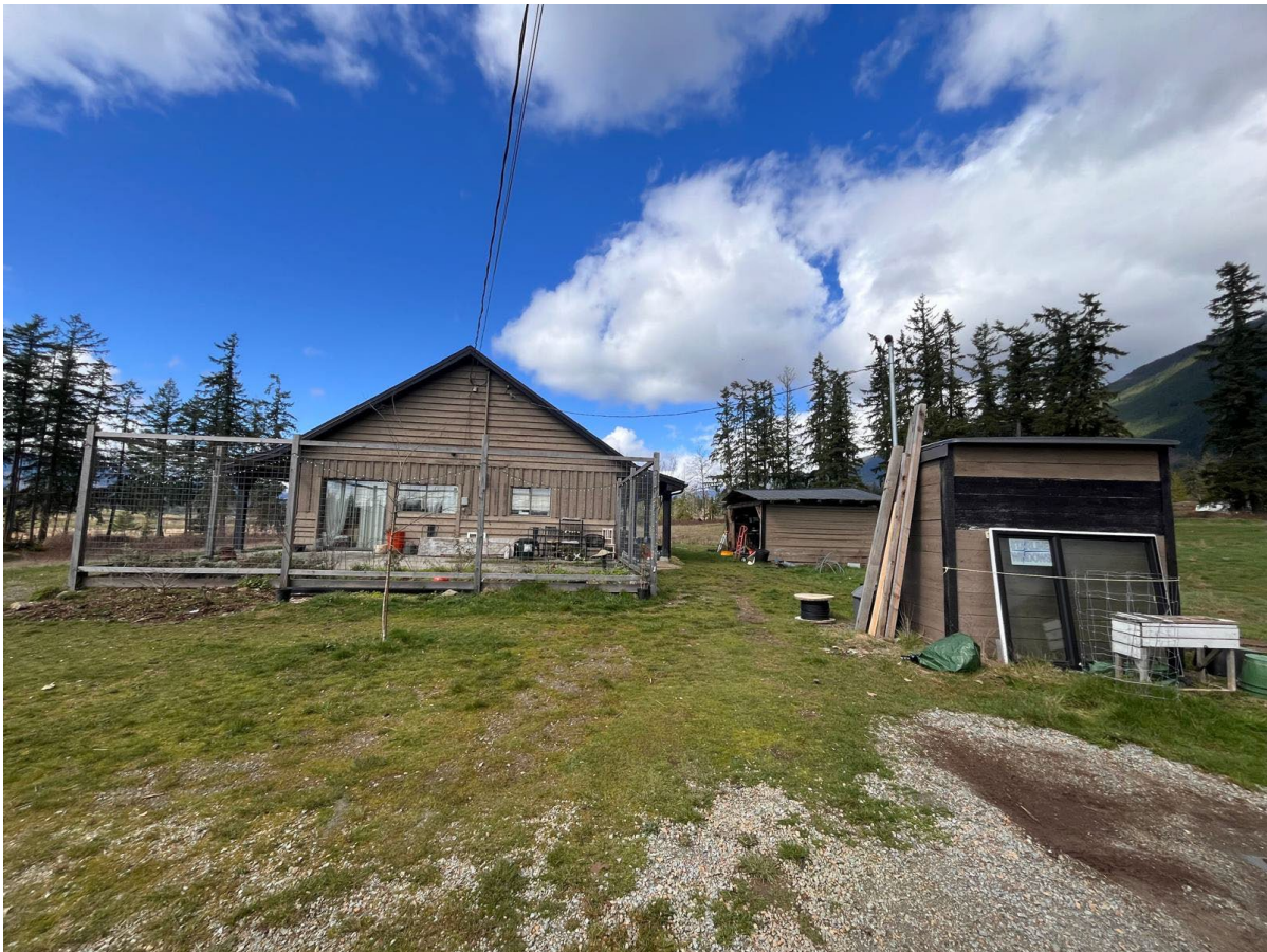
Existing dwelling unit and accessory buildings via Bryson Rd
