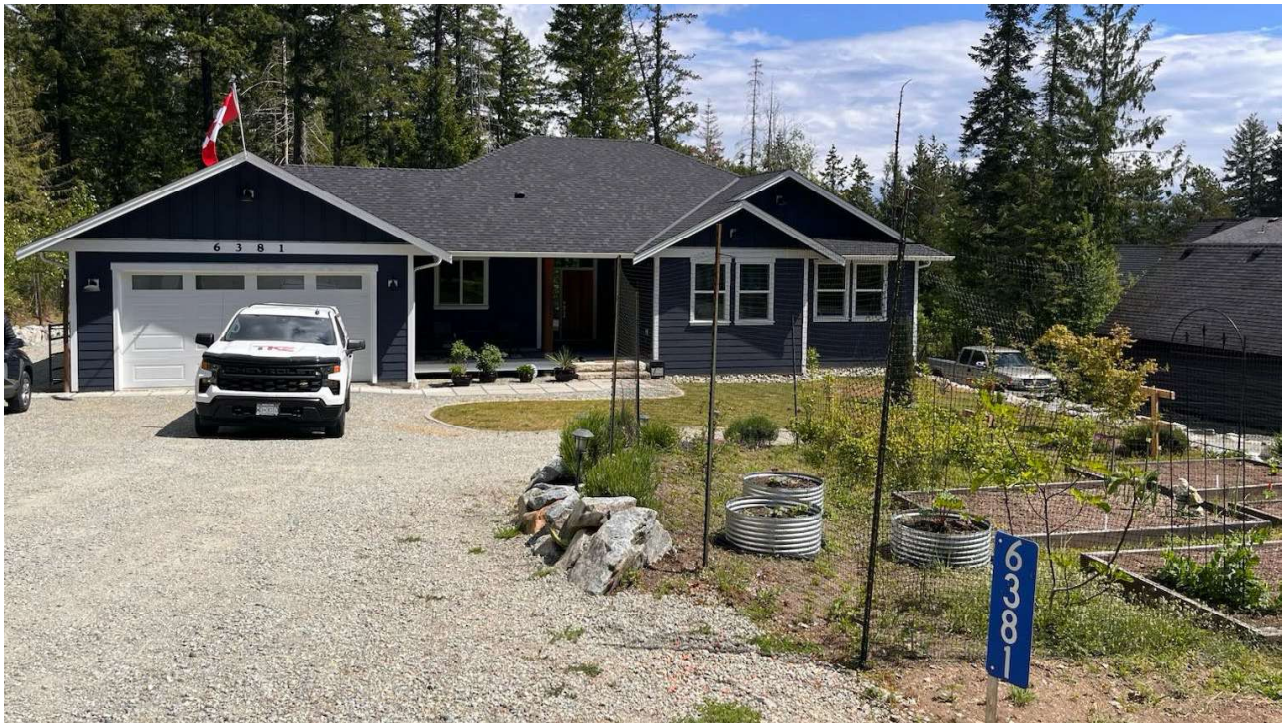
Front façade of the property looking east
