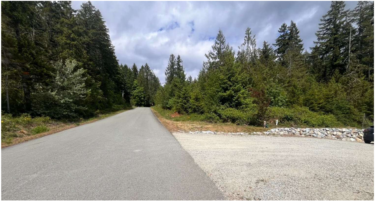
Existing driveway access from Salal Road
