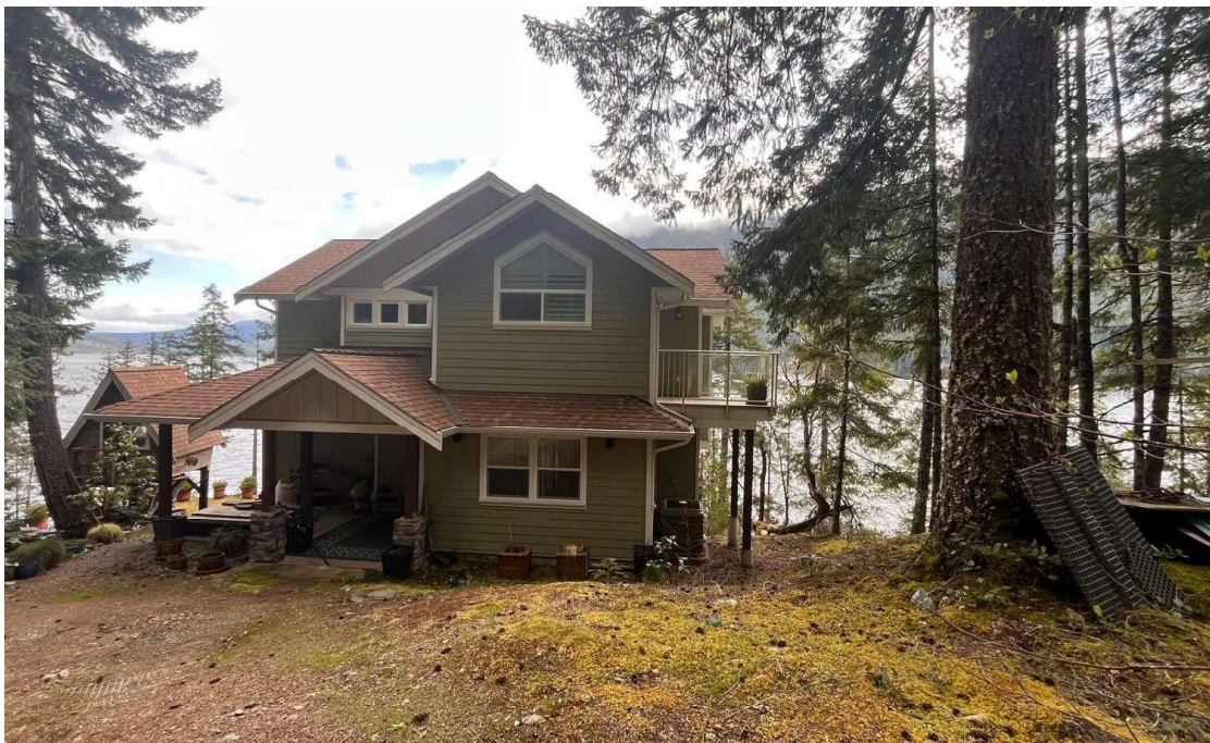
Existing dwelling unit and accessory building
