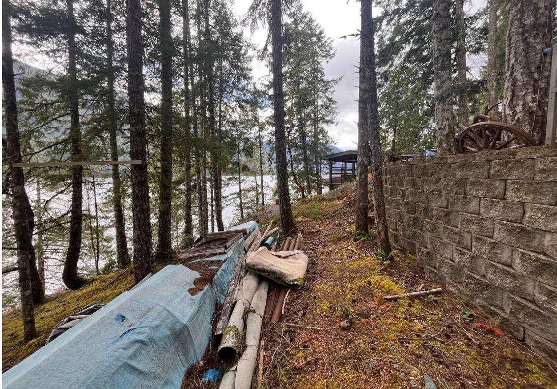
Site of proposed accessory building showing existing retaining wall
