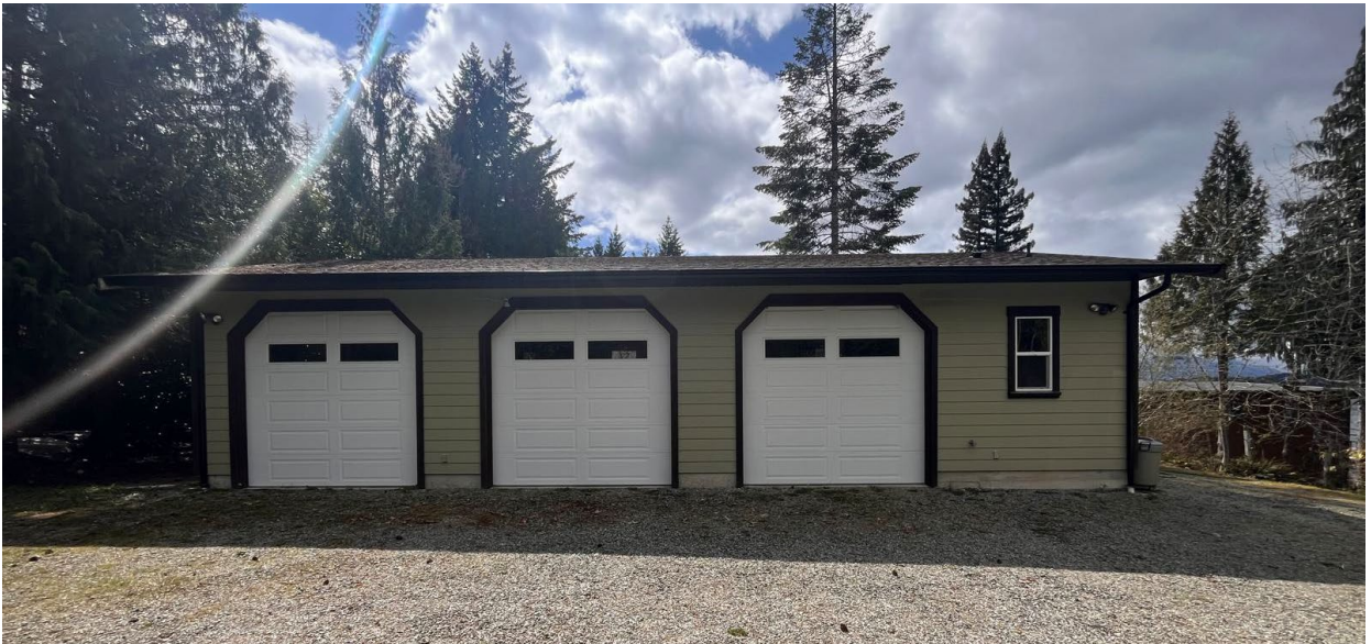
Existing garage structure
