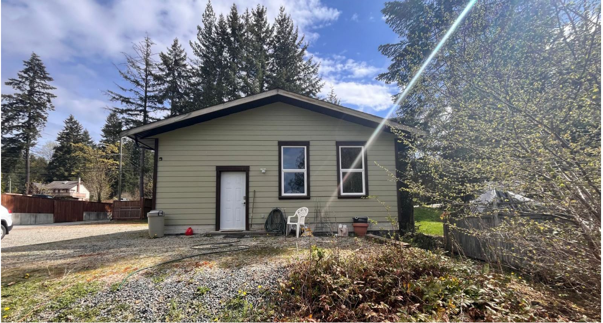
Existing garage structure with a 9 ft south side yard setback
