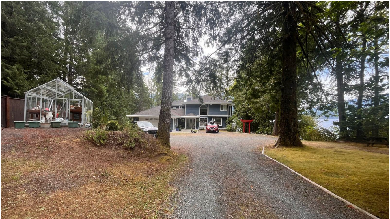
Existing Single-family dwelling on the property
