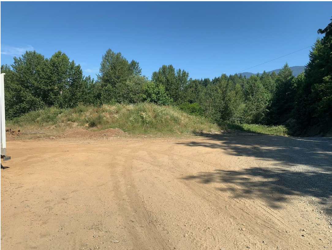
Upper bench area looking north toward the existing driveway. This area will be re-graded for the campground
