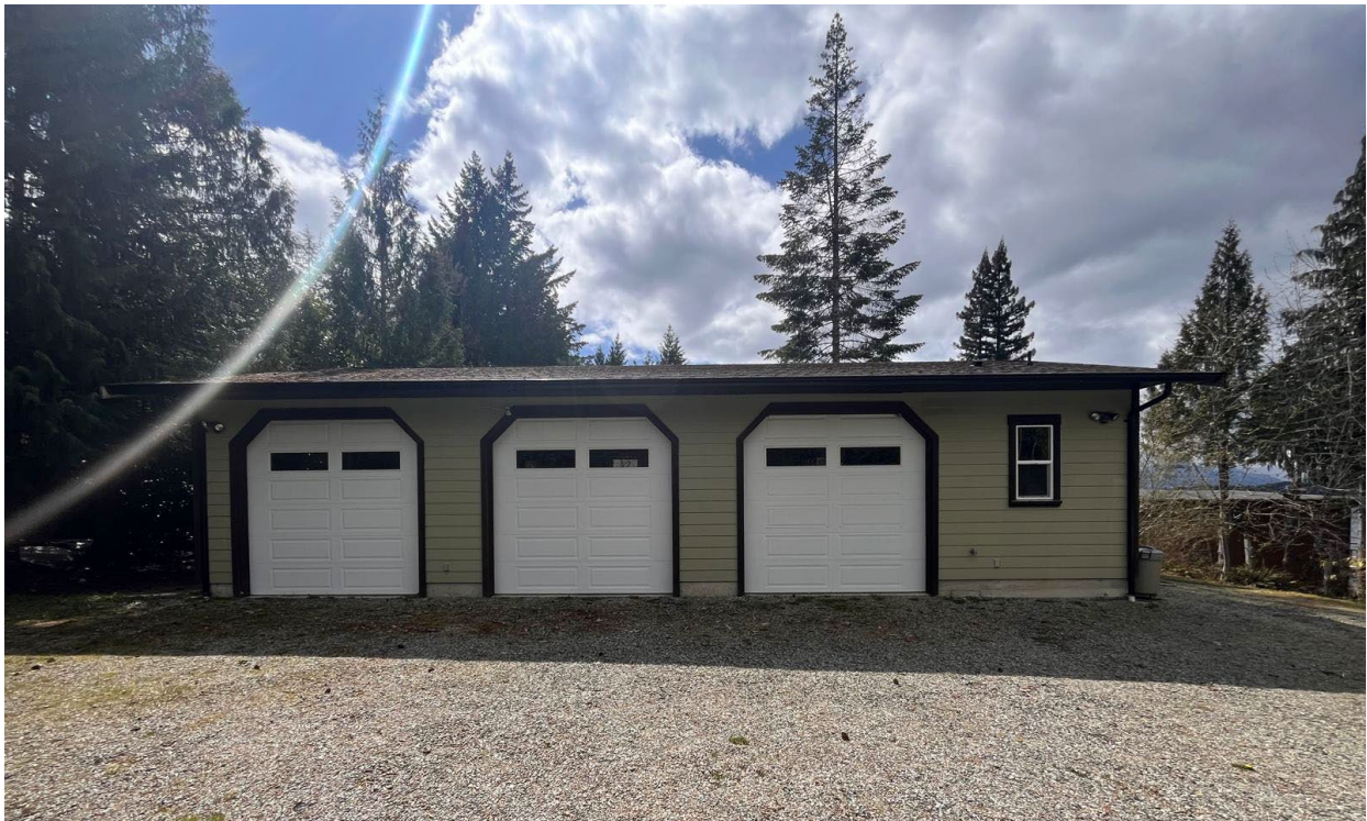
Existing garage structure
