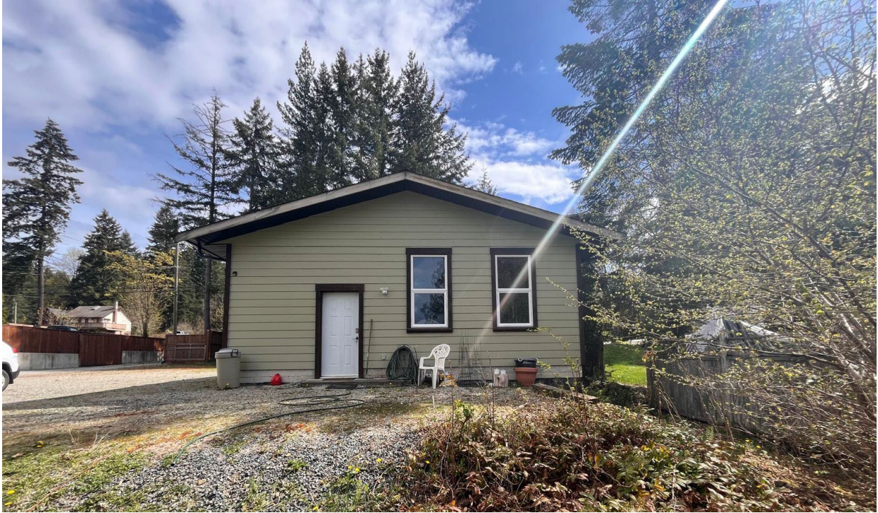
Existing garage structure with a 9 ft south side yard setback
