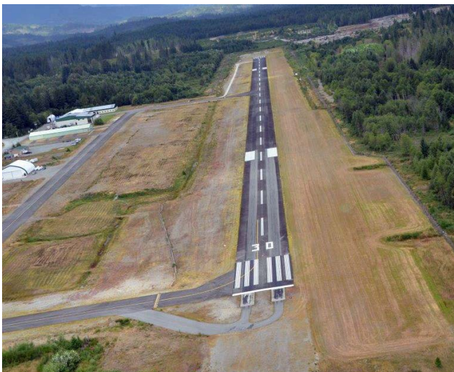
AVRA Prior to Expansion
