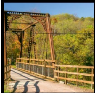
VISTA Bollman Bridge
