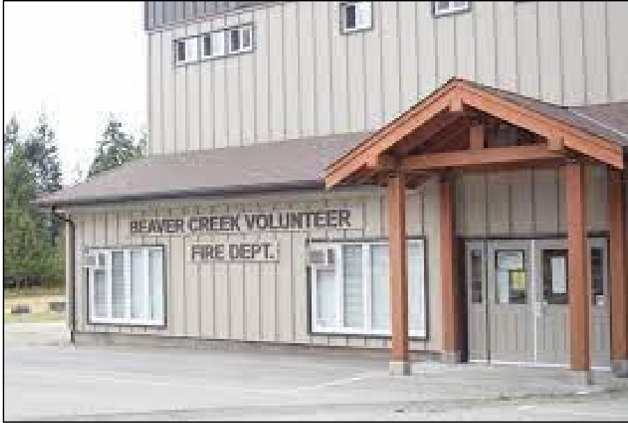
Figure 8: Beaver Creek, Hall 1 - Office Entrance
