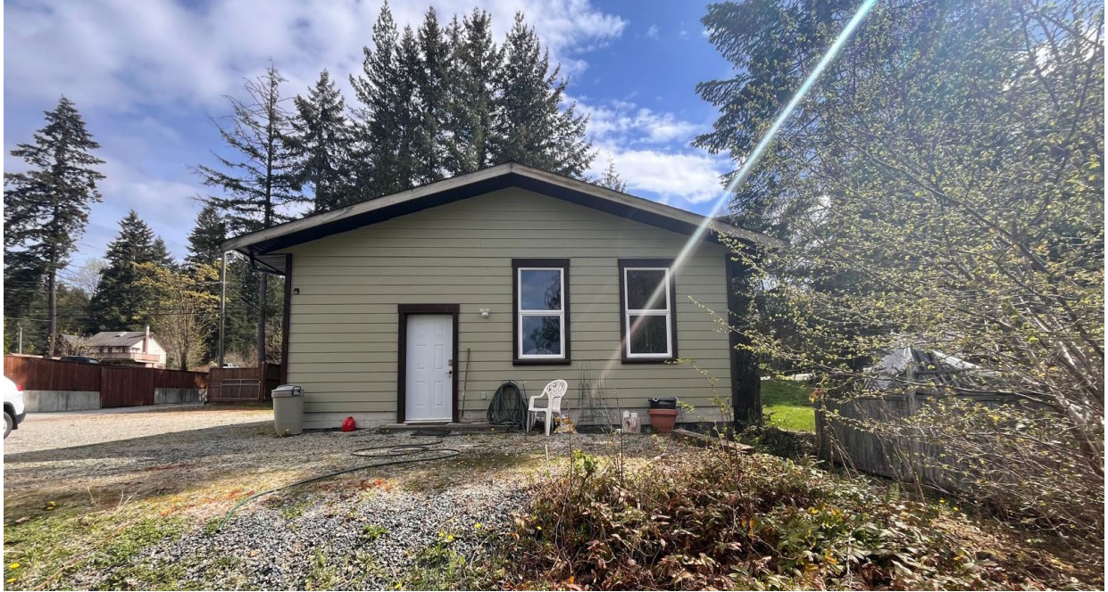
Existing garage structure with a 9 ft south side yard setback
