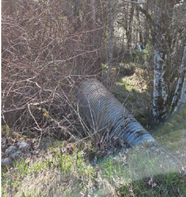
Exhibit 5. this pipe face to my farm, and creek water from this pipe flooding my land every year. Although it is located at property 450.
