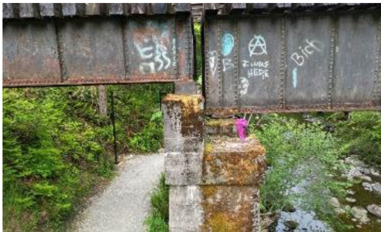
Figure 3-63: Bridge at Mile 37.1 – Pier 2 Foundation Minor Scour
