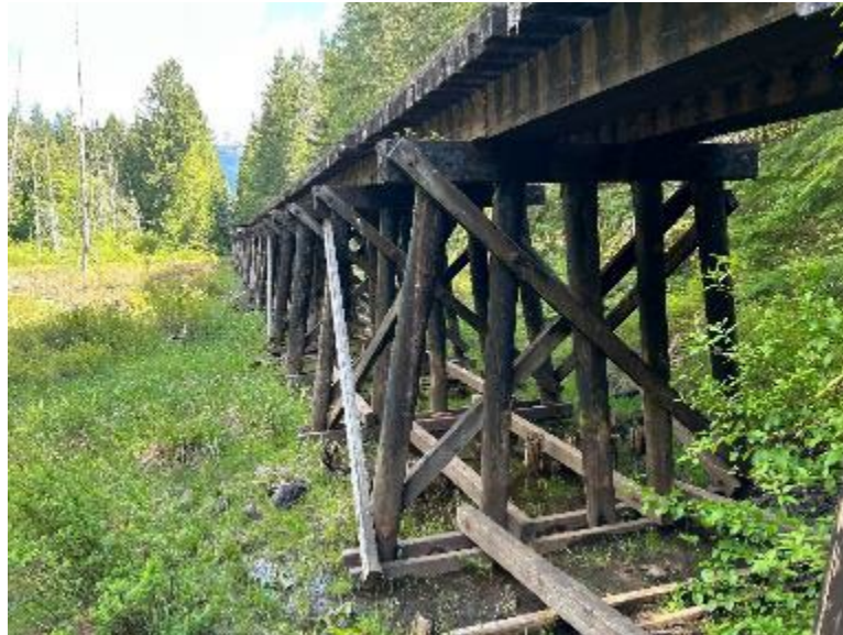
Figure 3-40: Bridge at Mile 21.8 – Under Side View Looking East
