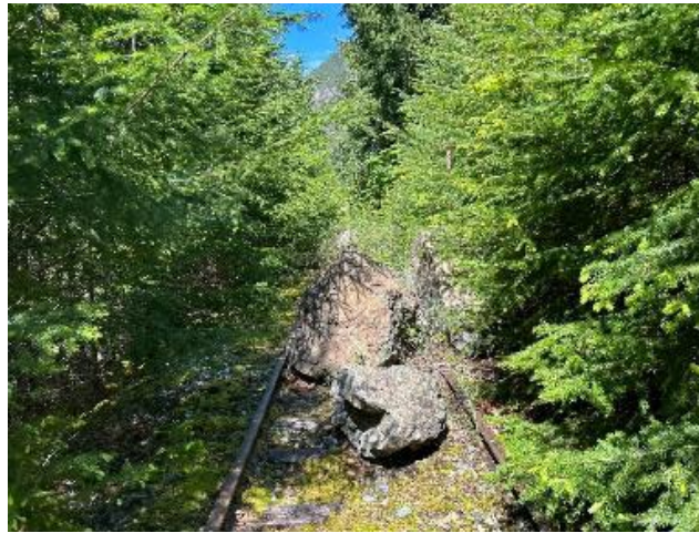
Figure 2-7: Segment 2 – Rockslide Mile 14.8
