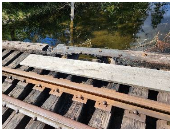
Figure 3-43: Bridge at Mile 22.1 – Fire Damage
