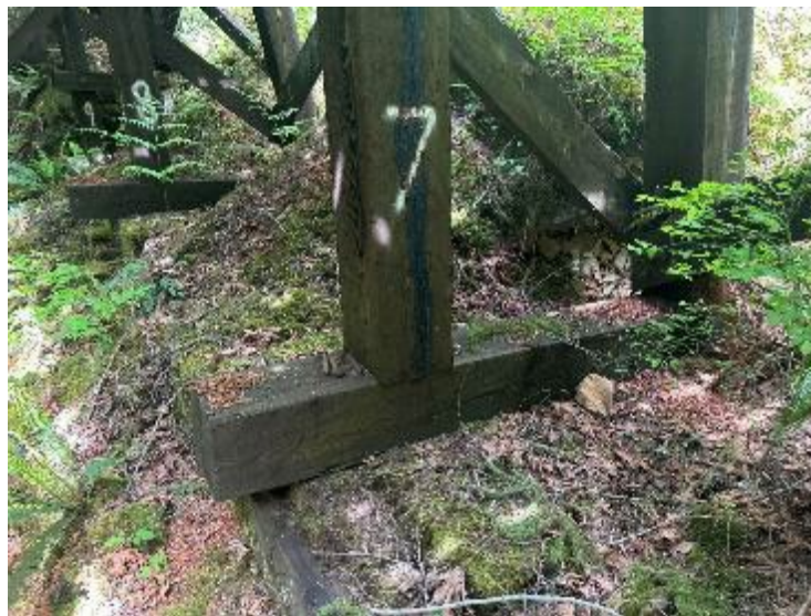
Figure 3-55: Bridge at Mile 29.9 – Decayed Mud Sills – Post 3, Bent 7
