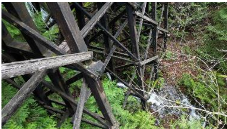
Figure 3-24: Bridge at Mile 17.5 – Center Interior Bents and Creek View
