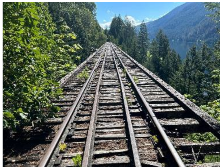
Figure 3-18: Bridge at Mile 14.6 – Deck View Looking East
