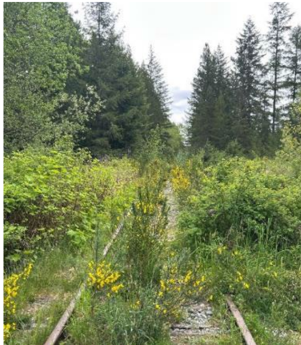
Figure 2-2: Segment 1 - Typical Track Roadbed
