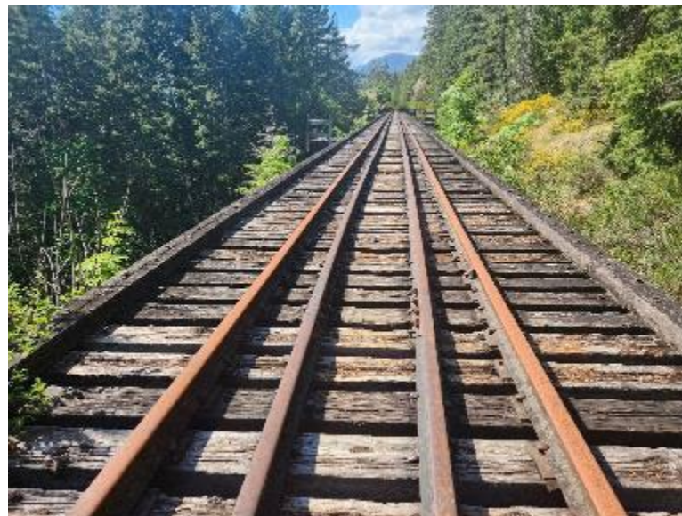
Figure 3-46: Bridge at Mile 25.0 – Deck View Looking West
