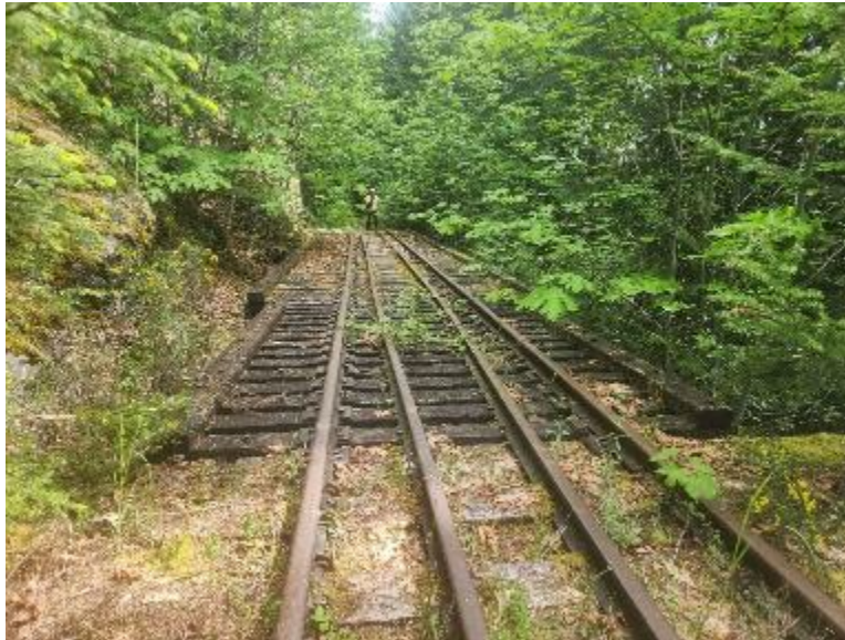
Figure 3-51: Bridge at Mile 28.9 – Deck View Looking East
