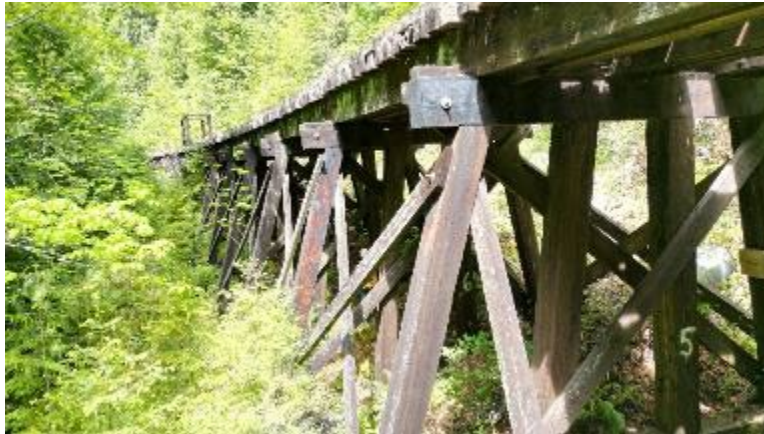
Figure 3-55: Bridge at Mile 29.9 – Decayed Mud Sills – Post 3, Bent 7
