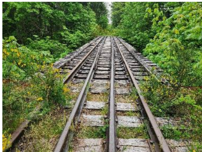
Figure 3-2: Bridge at Mile 4.7 – Deck View
