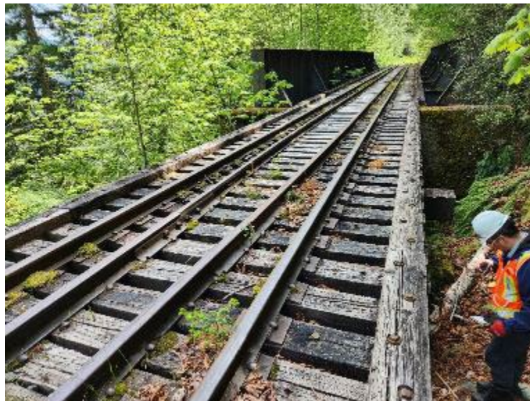
Figure 3-29: Bridge at Mile 18.8 – Deck View Looking West
