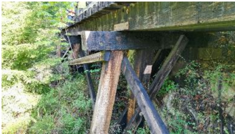
Figure 3-13: Bridge at Mile 13.8 – Typical Bent Cap View Looking West
