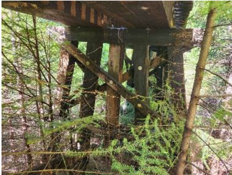
Figure 3-16: Bridge at Mile 14.0 – Typical Bent Frame
