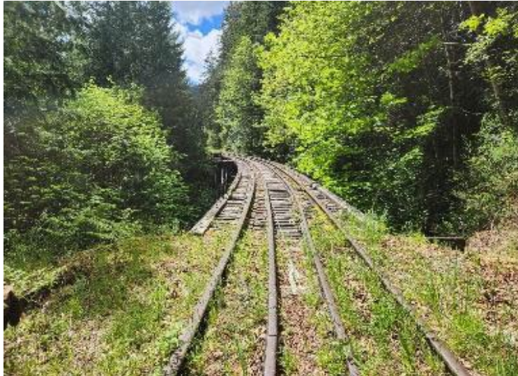
Figure 3-23: Bridge at Mile 17.5 – Abutment View Looking East
