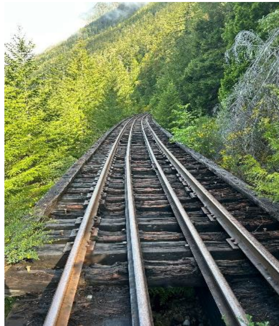
Figure 3-8: Bridge at Mile 13.7 – Deck View Looking West
