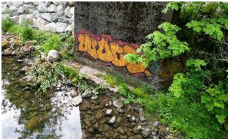
Figure 3-63: Bridge at Mile 37.1 – Pier 2 Foundation Minor Scour
