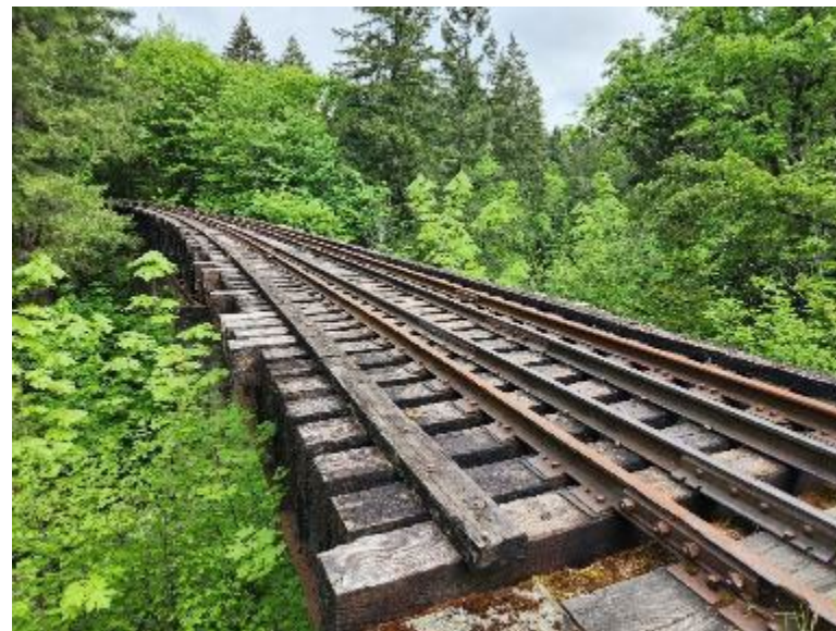
Figure 3-57: Bridge at Mile 36.5 – Deck View Looking East
