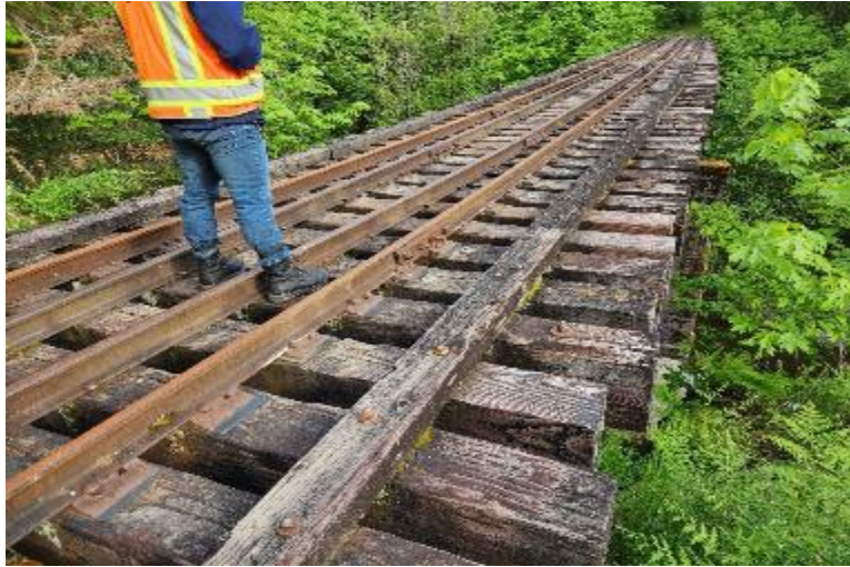
Figure 3-62: Bridge at Mile 37.1 – Pier View
