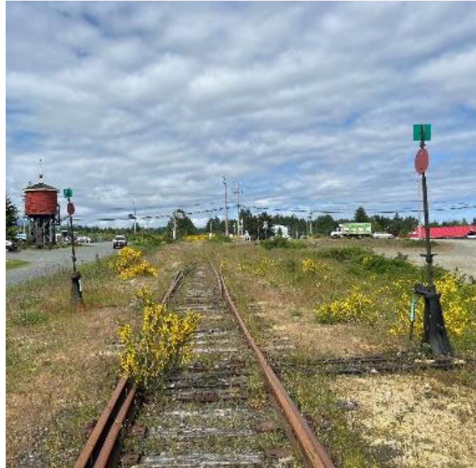
Figure 2-5: Segment 1 – Turnout Mile 0.03
