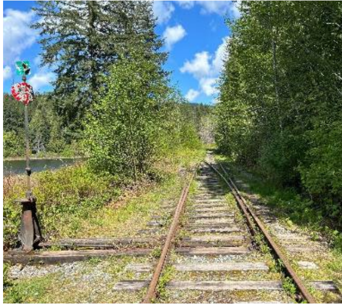
Figure 2-11: Segment 2 – Turnout Mile 21.95
