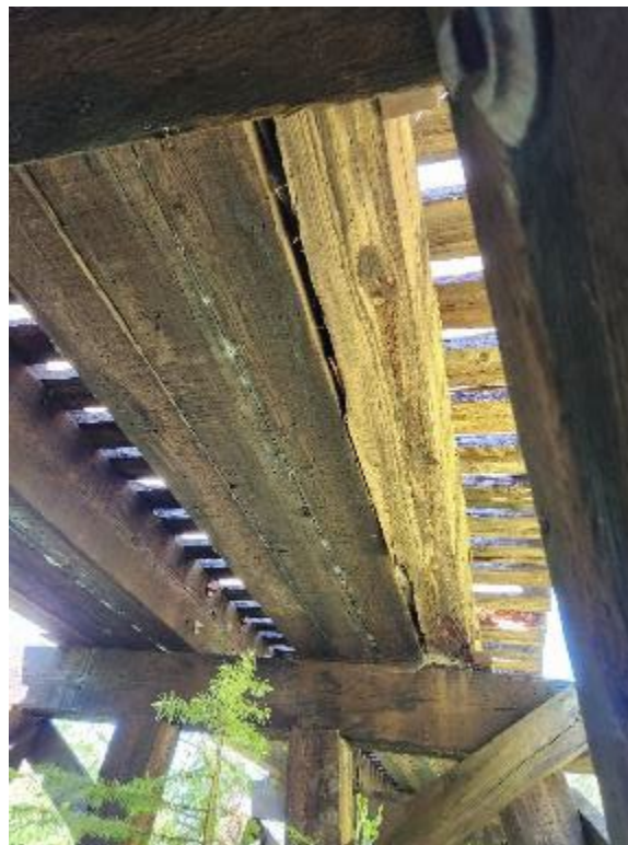
Figure 3-20: Bridge at Mile 14.6 – Stringer Chord Splitting
