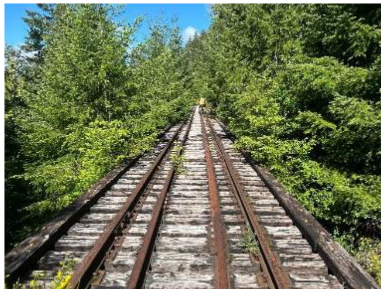
Figure 3-15: Bridge at Mile 14.0 – Deck View Looking West
