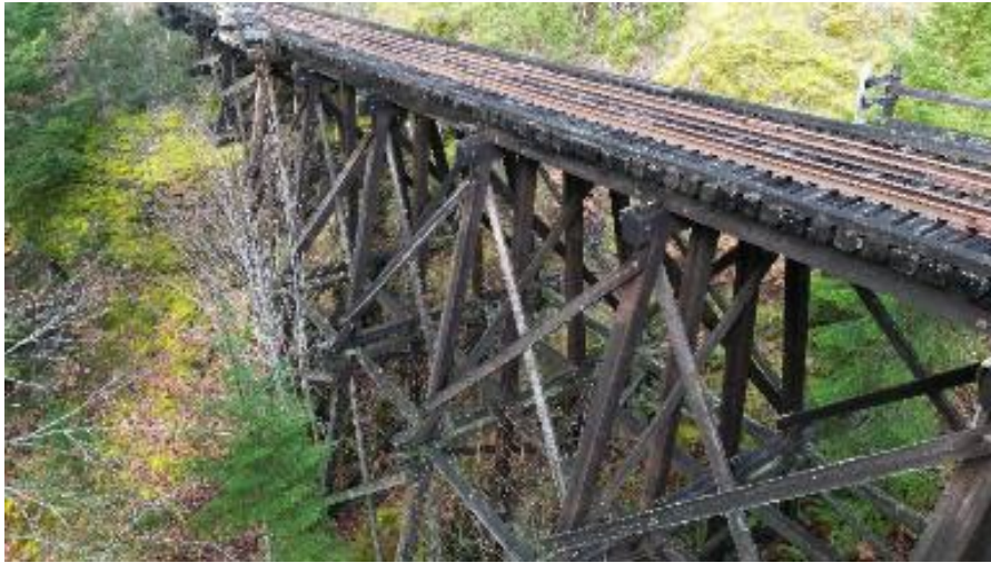
Figure 3-47: Bridge at Mile 25 – South Elevation
