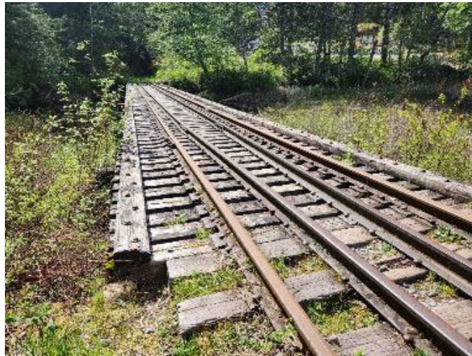
Figure 3-43: Bridge at Mile 22.1 – Fire Damage
