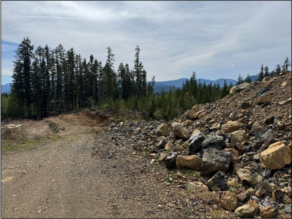
Pictures #7-9 – gravel pit in southwest corner of property
