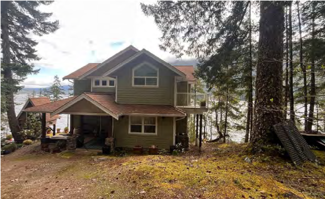
Existing dwelling unit and accessory building
