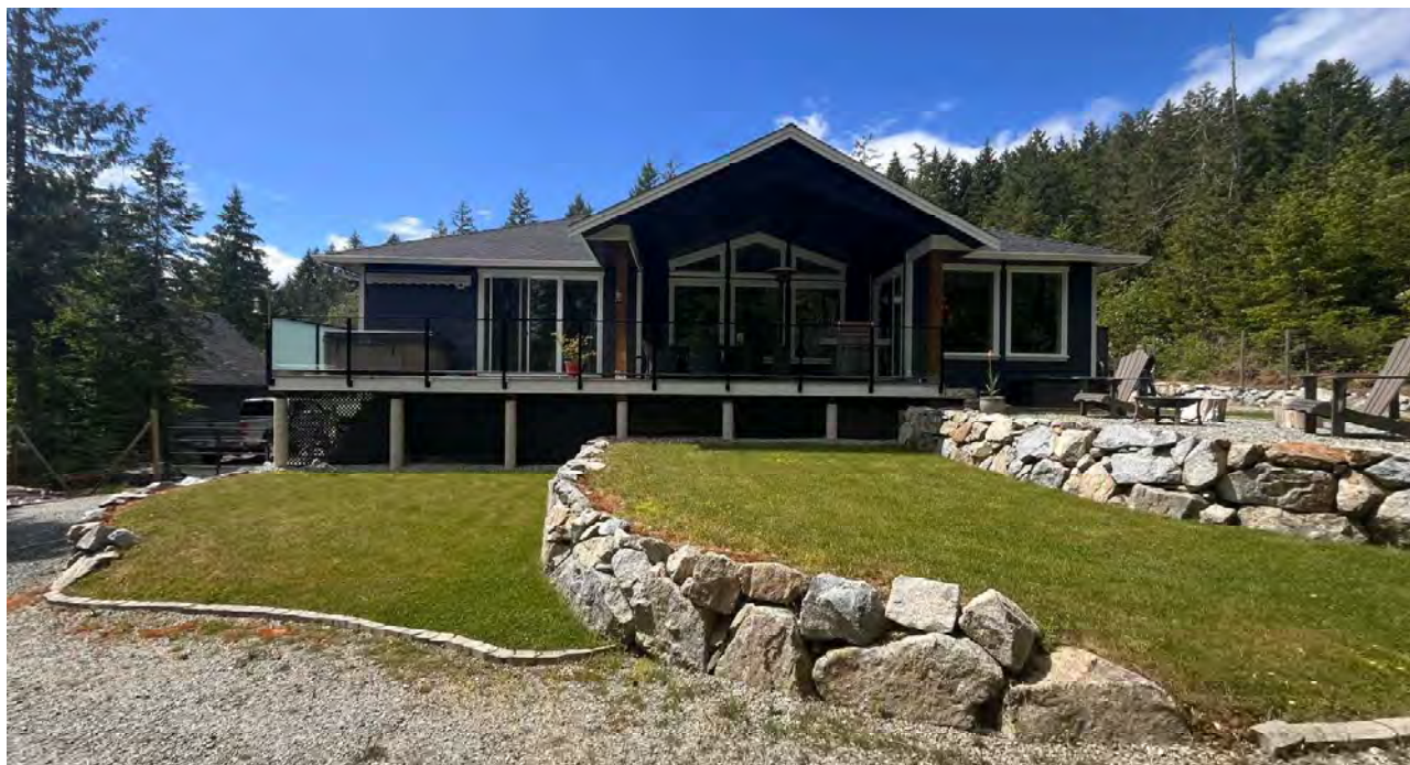
Back façade of the property looking west
