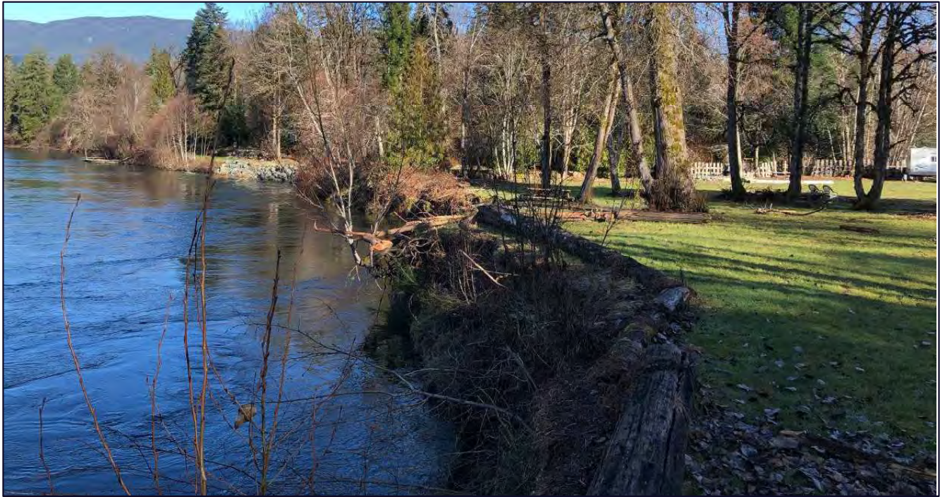
Figure 2.6.2 – Typical Foreshore Conditions (View looking North)
