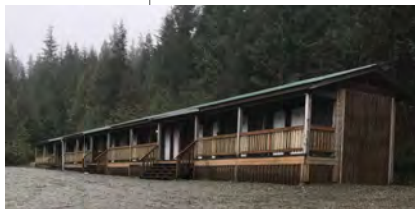
② VIEW OF BUILDING 1 FROM SW CORNER OF SITE
