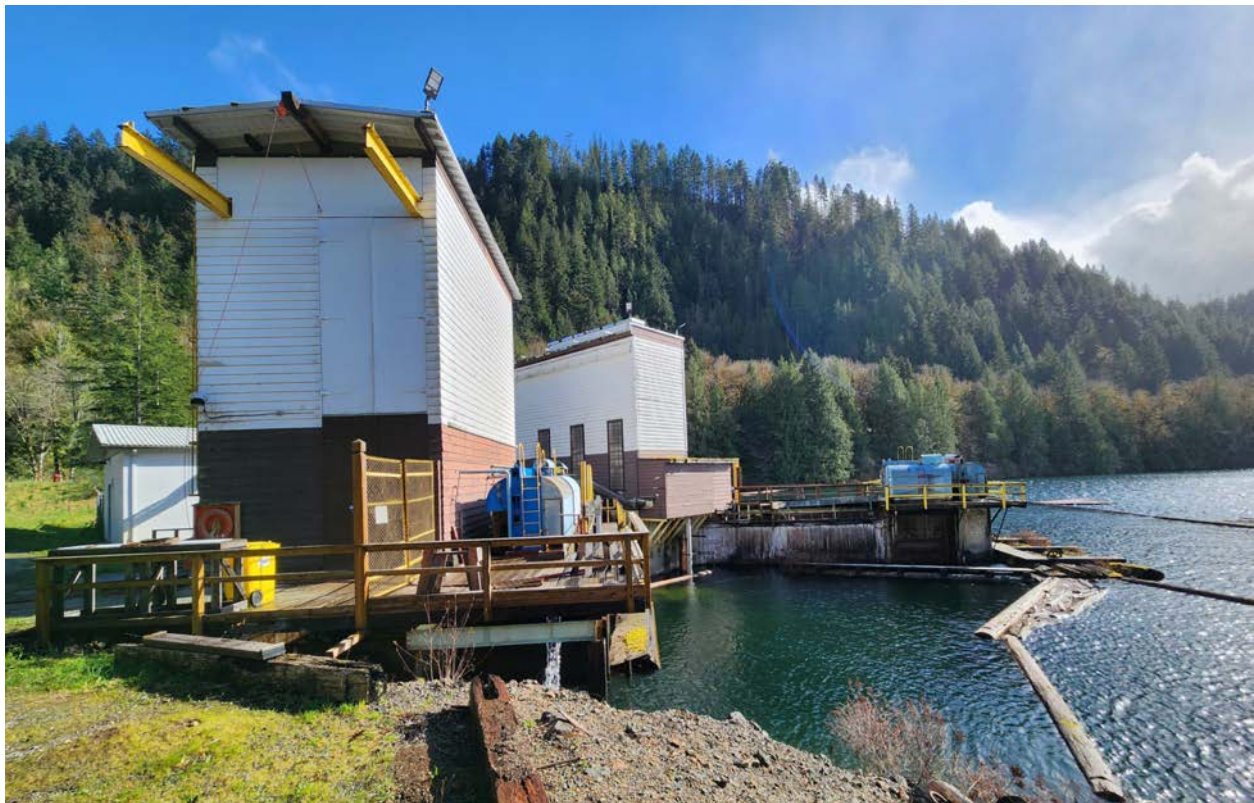
Figure 14. Water intake infrastructure on Sproat Lake owned by Domtar Industries.
