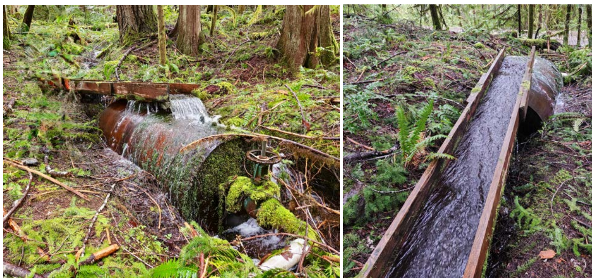
Figure 19a and 19b. Water seepage and collection at the bottom of the Beaufort Mountain Range.
