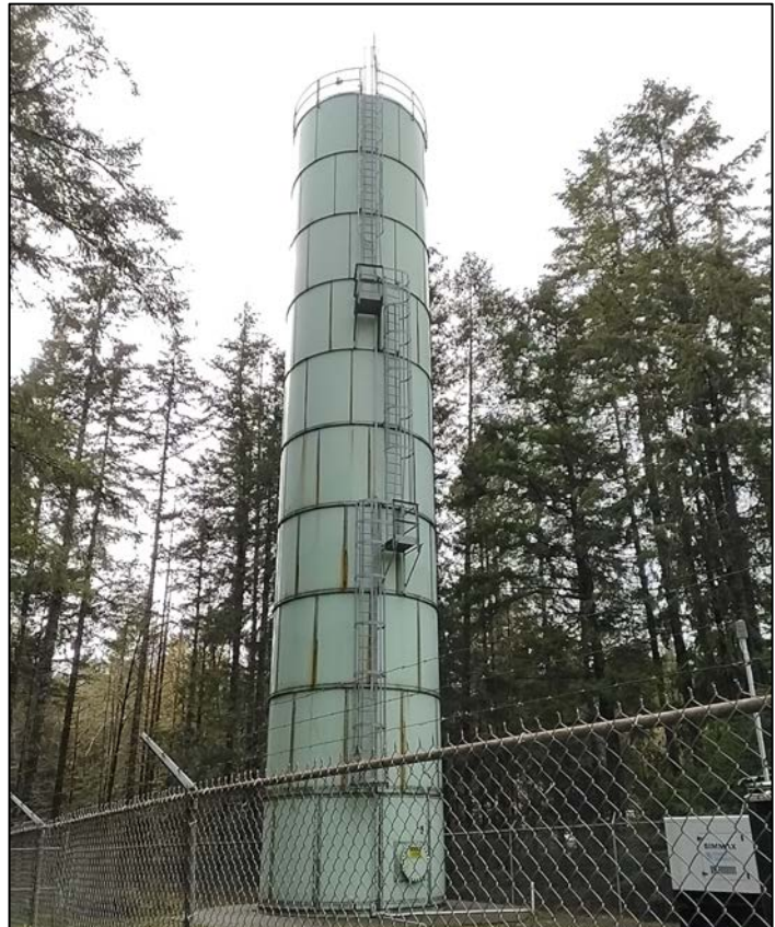
Figure 28. Steel water reservoir located on Beaver Creek Road.
