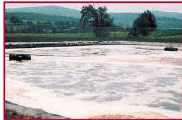
Aerated Lagoon (Source – www.integrityagsystems.com )
