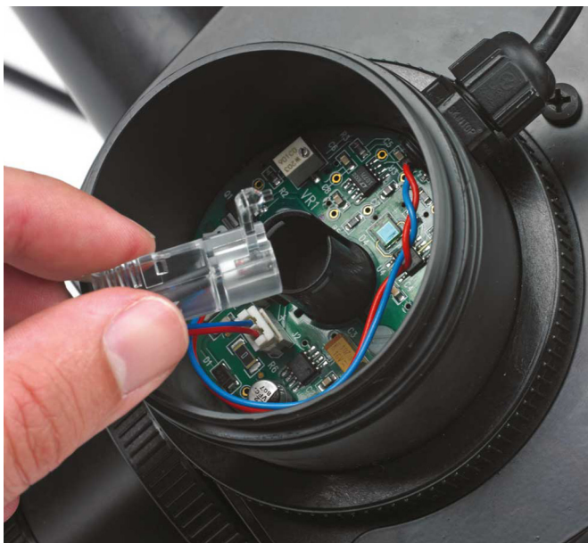
Fig. 6: Replacing the light source
