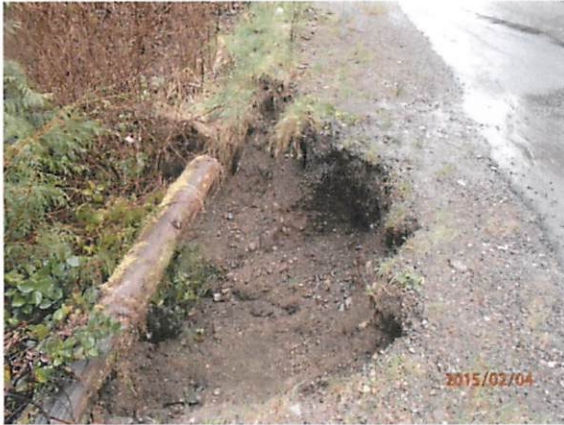
Photo 5: Outlet of Creek 6 showing collapsed roadway
