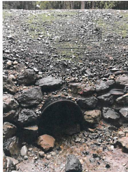
Photo 4: Completed culvert installation on Creek 4
