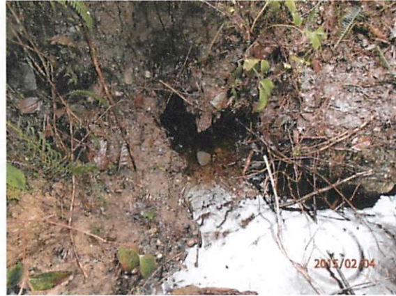
Photo 6: Creek 6 culvert inlet before restoration
