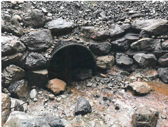
Photo 3: Inlet of newly installed culvert on Creek 4
