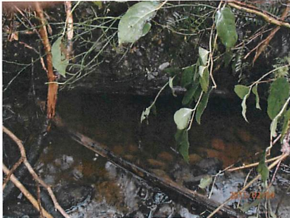
Photo 1: Outlet of Creek 4 culvert before replacement
