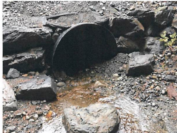
Photo 8: Creek 6 culvert after installation completed
