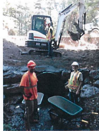
Photo 2: Creek 4 after culvert installation during embedment
