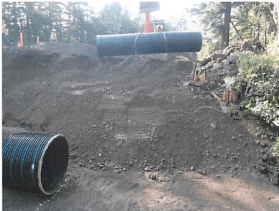
Photo 7: Creek 6 culvert installation during construction works
