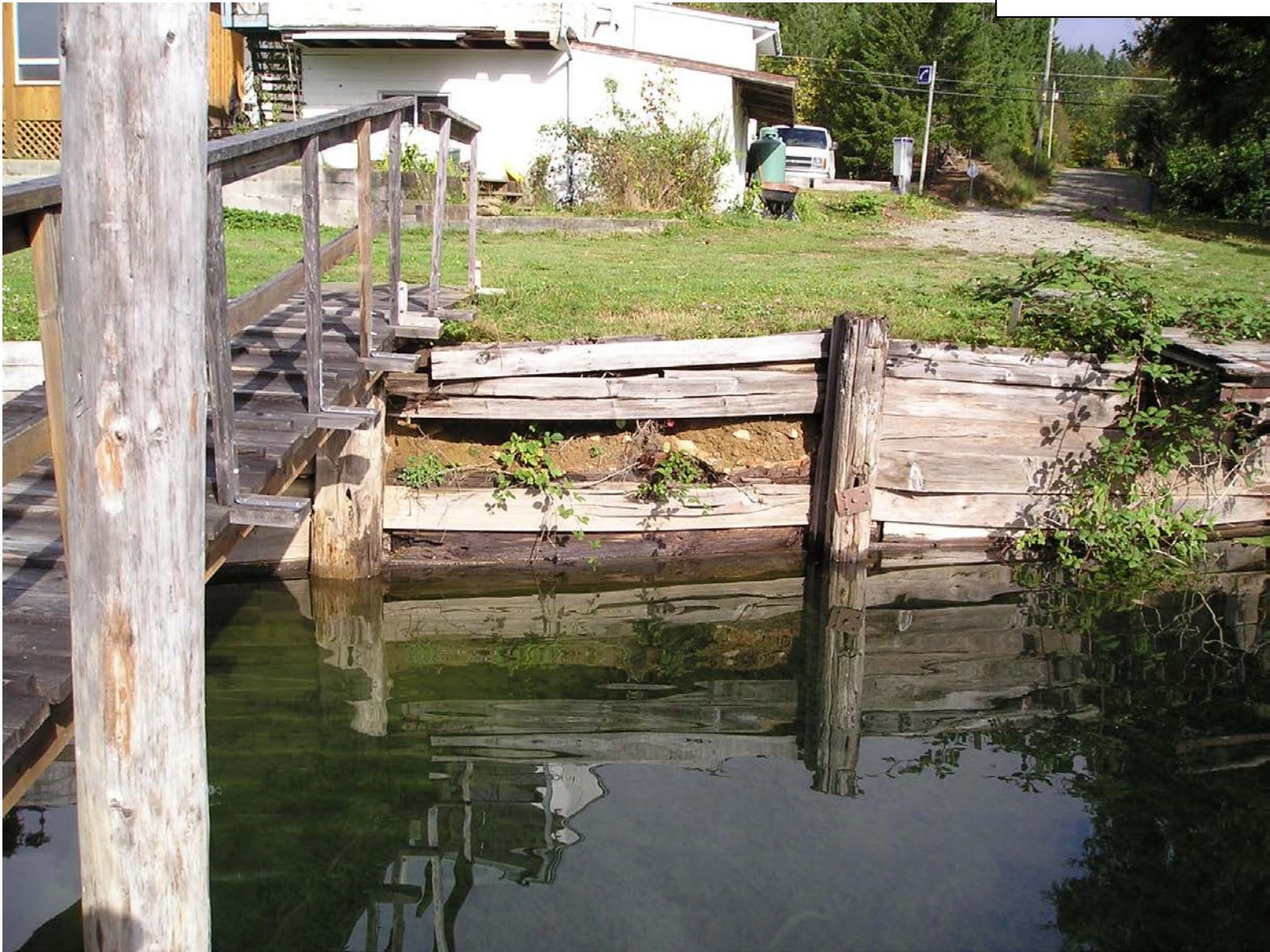
Shored up collapsed embankments
