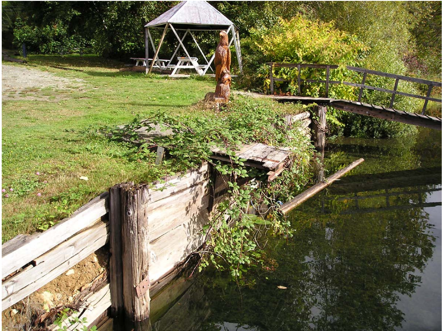
Repaired/replaced unsafe walkways and ramps
