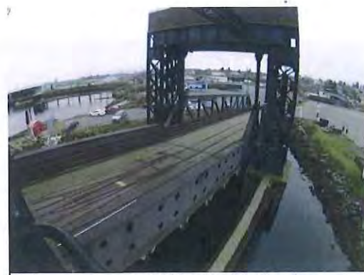
Rail marine ramp at Wellcox Yard in Nanaimo.
