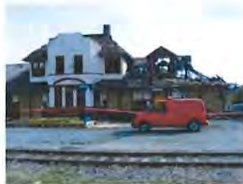
Before (following the fire of 2007)
