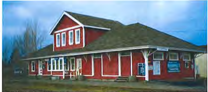
The Courtenay Rotary Club recently completed critical upgrades at the Courtenay train station, including a new roof and upper siding. The ICF is now working to partner with another local organization to complete interior renovations and attract new tenants.
