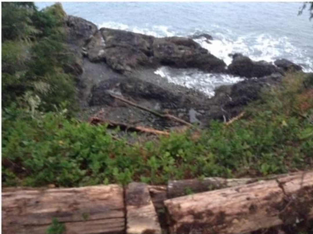
2.) From top of bank looking at existing cleared area
