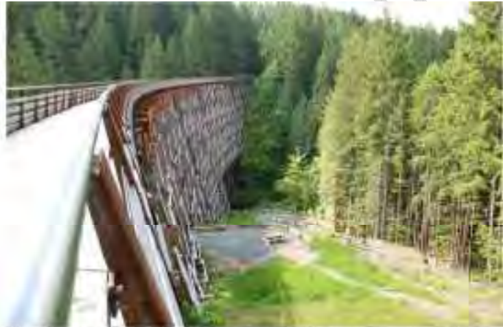
The Historic Kinsal Trestle is one of eight trestles along the Cowichan Valley Trail route. At 117 metres in length and standing 44 metres above the Kabinas River, it is one of the tallest free-standing and most spectacular timber rail trestle structures in the world. (Photo Credit / Source: Cowichan Valley Regional District)
