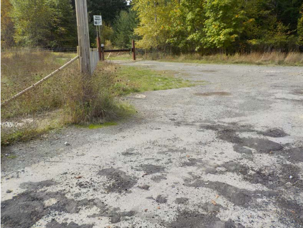
Figure 5: Pavement on Beaver Creek Road shoulder in front of former store.
