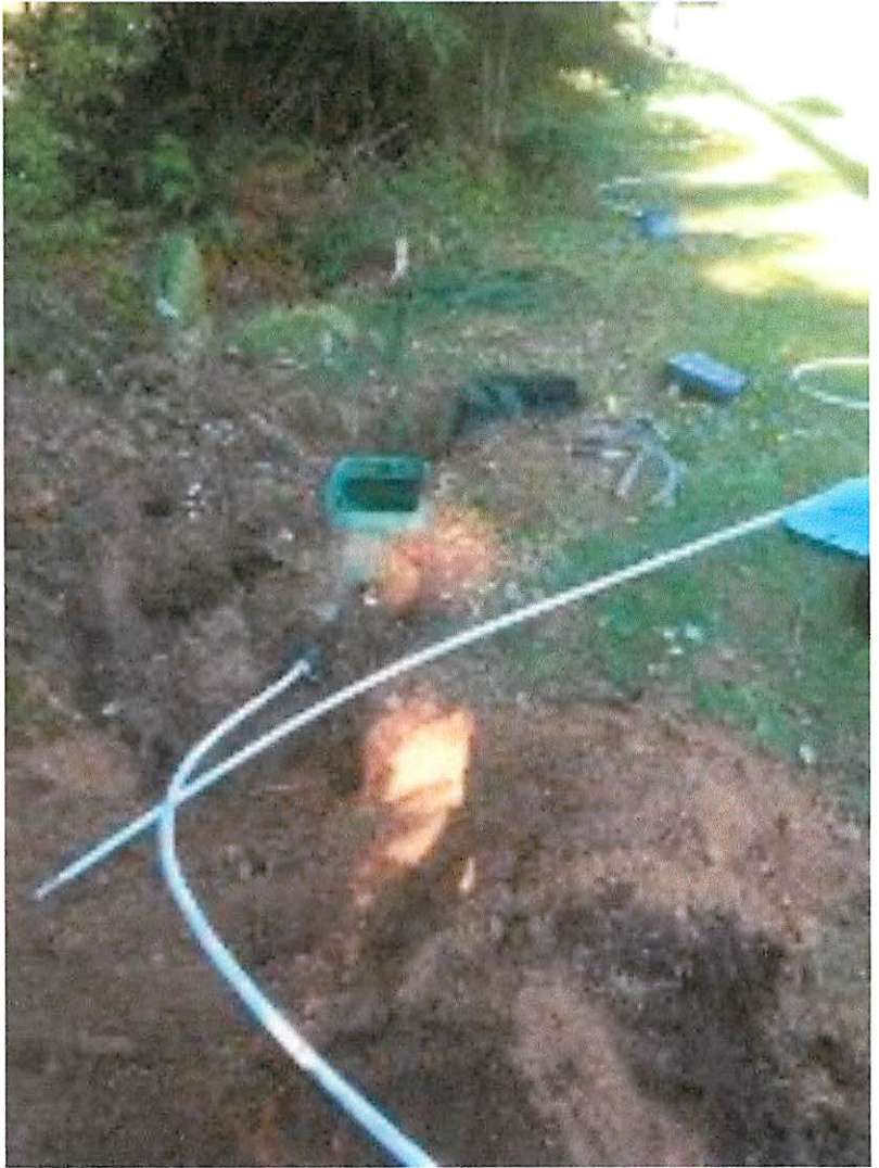
Another image of the temp. connection of the per to the old water main.
