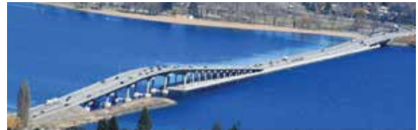
The five-lane William R. Bennett Bridge on Highway 97, completed in 2008, is the only crossing of Okanagan Lake. It serves the entire valley and directly connects Kelowna with West Kelowna.
