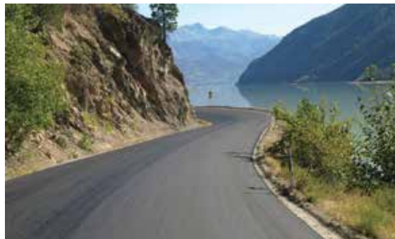
Side road paving near Lillooet
