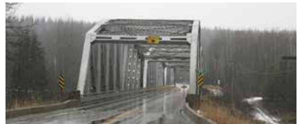
Parsnip Bridge, Highway 97
