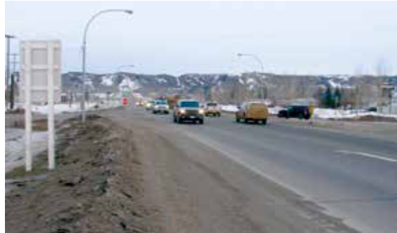
A new traffic signal in Taylor will be installed on the Alaska Highway at Pine Avenue in 2015.
