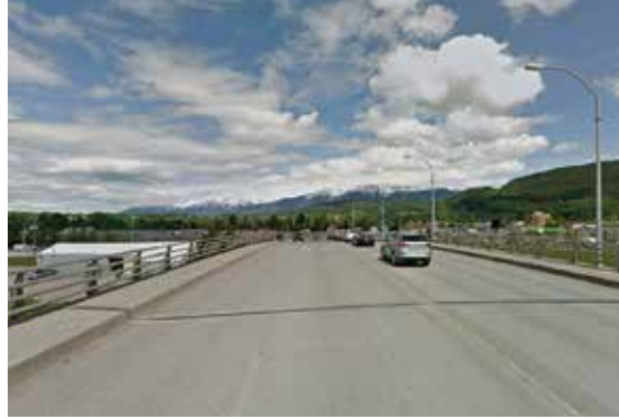
Sande Overpass bridge deck in Terrace will be resurfaced.
