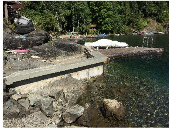
3) Existing patio footing
