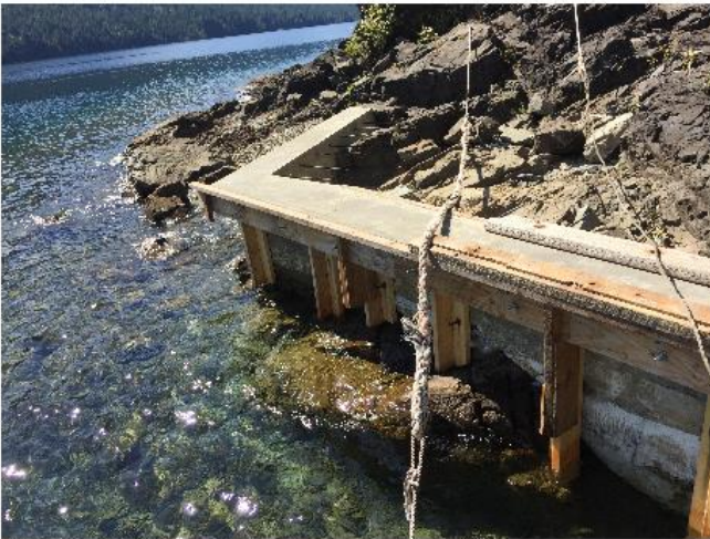
2) Existing patio footing on bedrock
