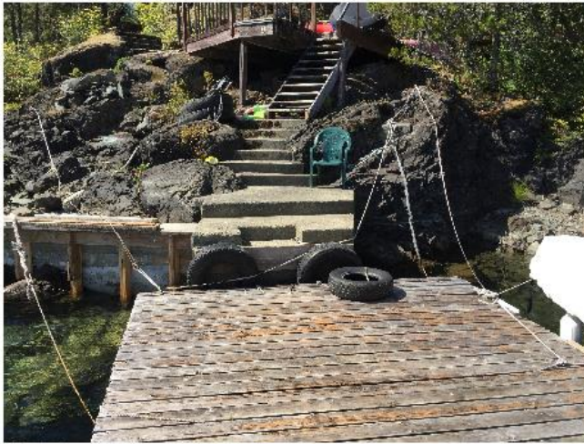
1) Existing stairway and patio footing
