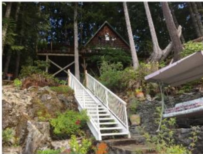
2.) Existing house looking upstream from lakeshore
