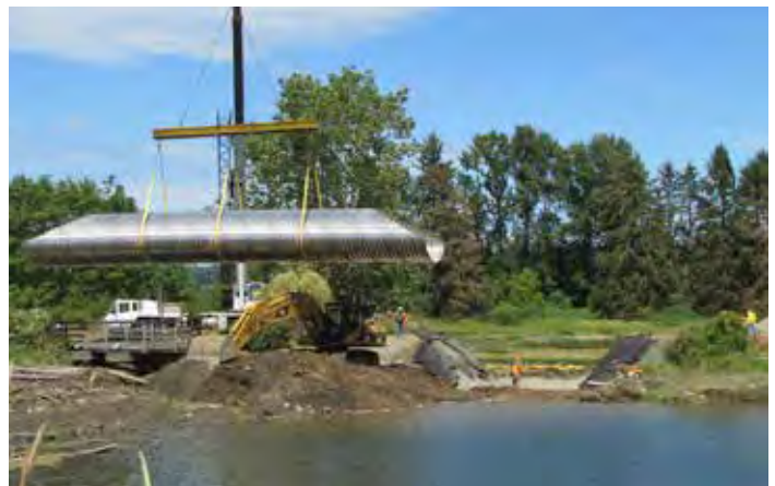
Large Culvert lifted into place at the Airport Marsh. Photo taken by Dan Bowen.
