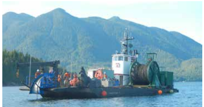
Crews lay cable in phase one of the Tofino to Ahousaht Reinforcement Project.
