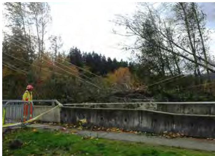
Cowichan Valley: A wire guard stands near low hanging lines to ensure public safety during storm events.
