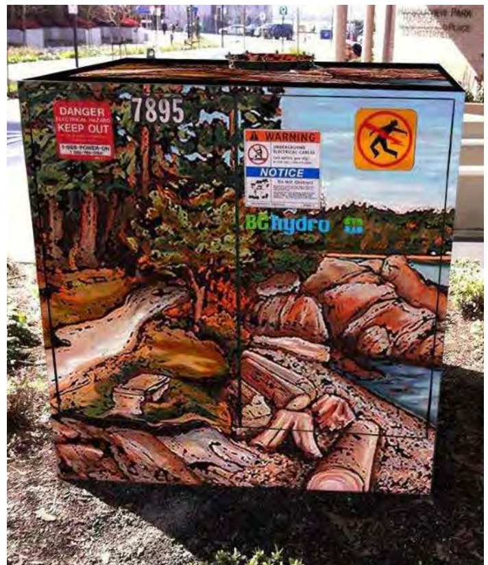
An example of a decorative wrapped pad-mount transformer in Richmond.
