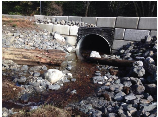
Figure 5: Newly installed aluminumized culvert on Maltby Creek
