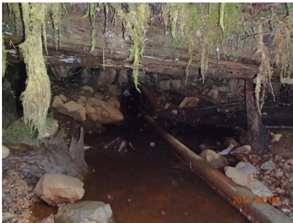
Figure 4: Outlet of culvert on Maltby Creek in English Cove – collapsing woodbox culvert with 600mm CSP
