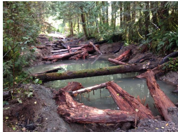
Figure 1: New off-channel habitat constructed on Creek 9 to allow for both over-wintering and summer refuge
