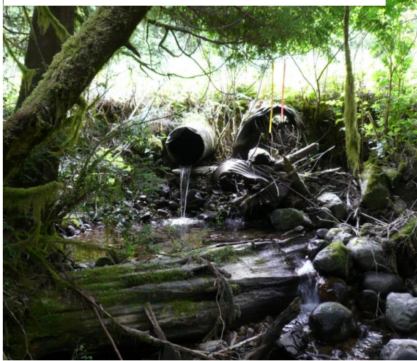
Figure 2: Hung and collapsed culvert on Creek 9 with CCW before construction
