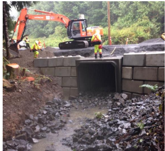
Figure 3: Newly installed 2.7m wide concrete box culvert on Creek 9 within CCW
