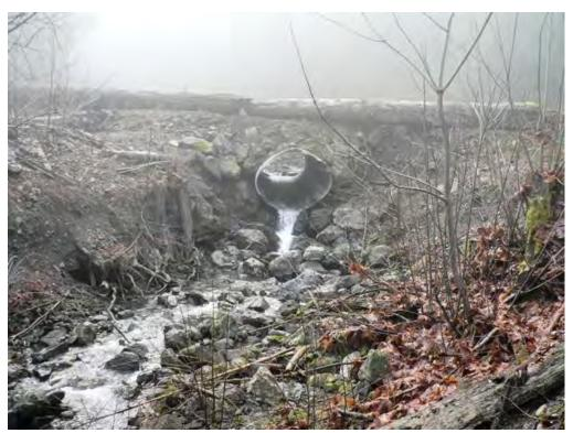
Photograph 2. View of perched culvert outlet on St. Dennis Creek.
