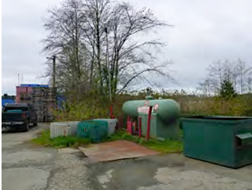
View to west depicting riparian zone on right (north) side of wharf approach. Note marginal storage of pallets and totes.
