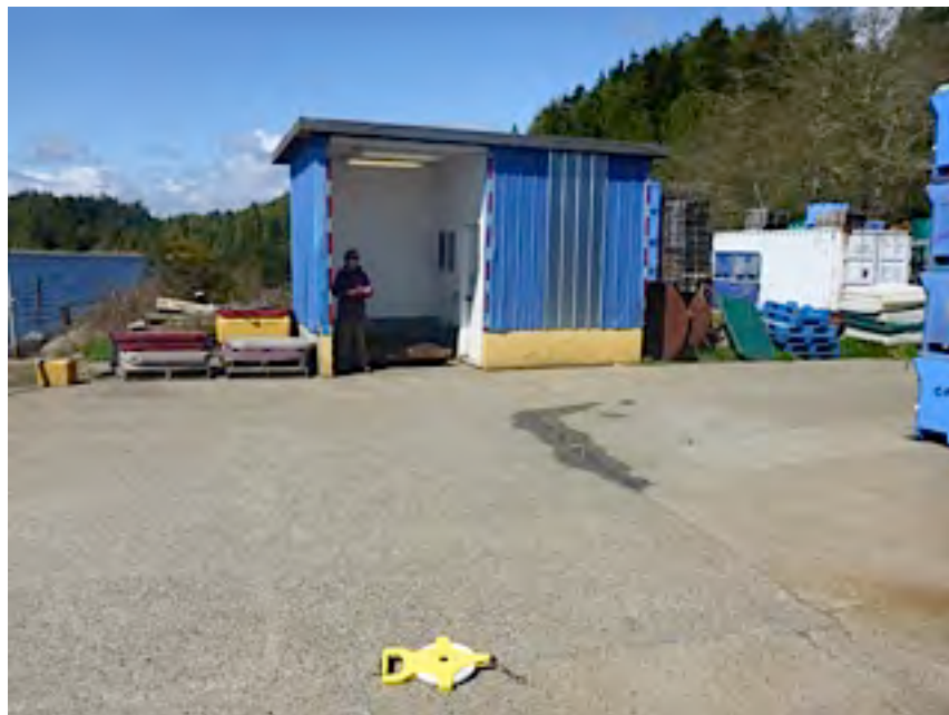
Photo 2. View north from SW corner of proposed ice plant location showing concrete pad & existing scale house.
