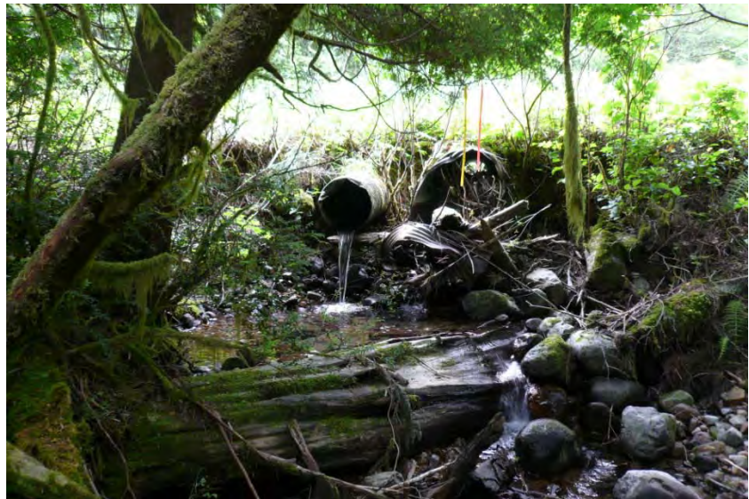
Figure 1 Conference Creek 9 culverts are hung impeding fish passage across highway 4 and access to valuable upstream habitat.
