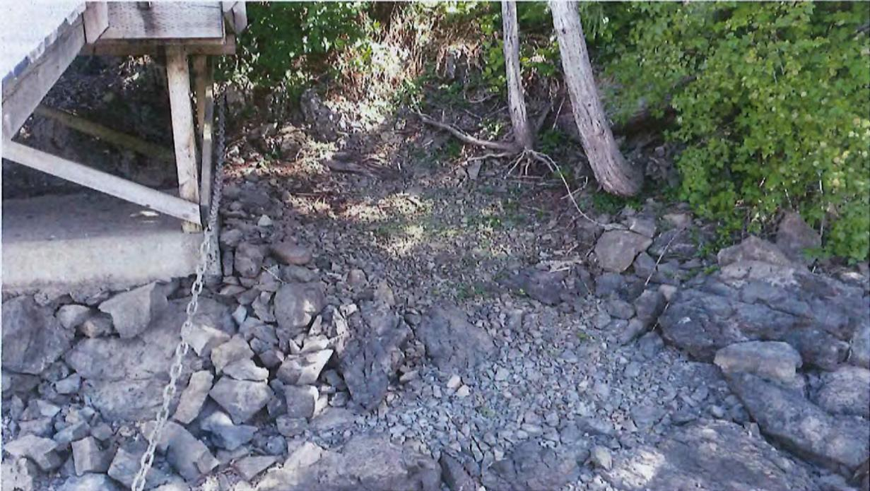
Showing location of Bedrock & Boulders at Lower Tram Landing next to Existing Stair Landing.
