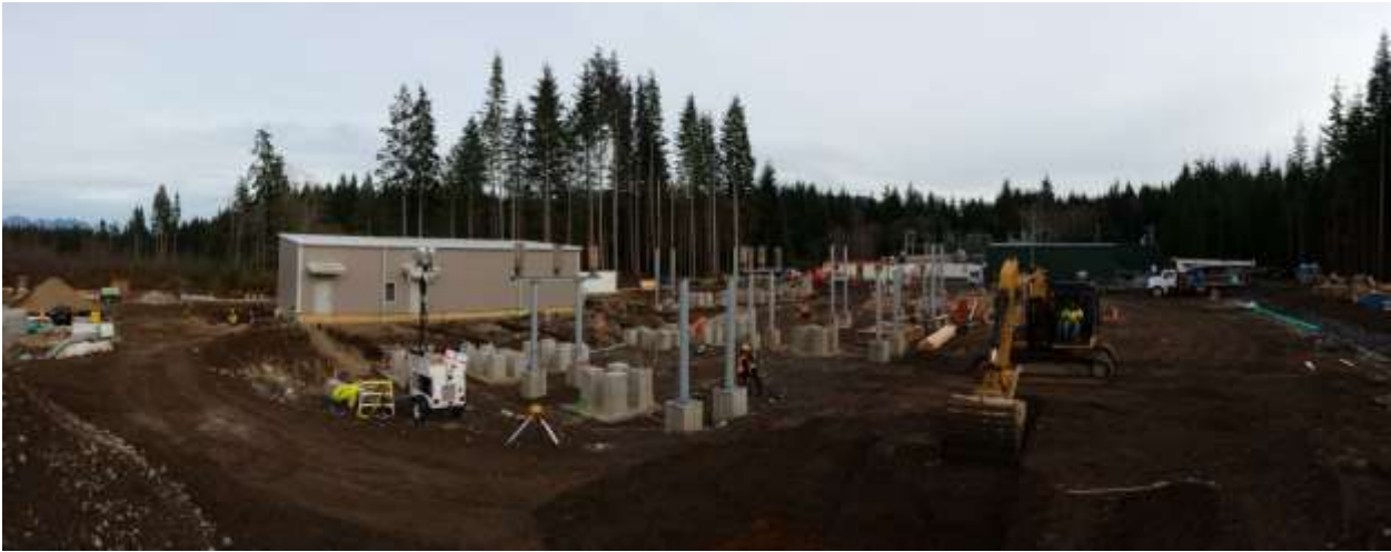
Long Beach substation – November 2014
