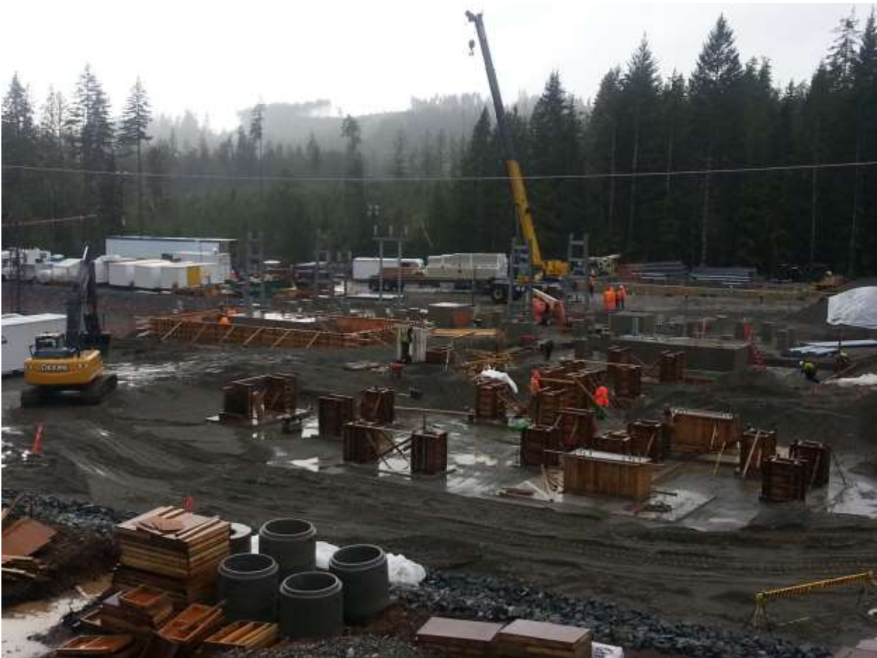
Great Central Lake substation – October 2014
