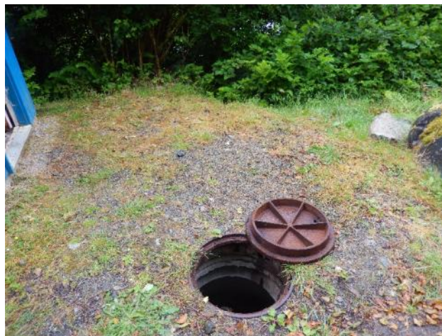
Figure 35: Chlorine injector vault (Grappler Road)
