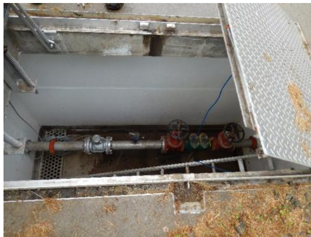
Figure 39: Coast Guard meter chamber
