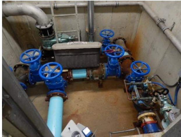
Figure 2: Beaver Creek north reservoir chemical injector room
