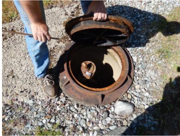
Figure 6: Stamp River air valve chamber
