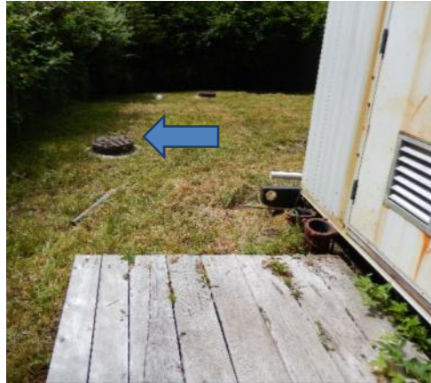
Figure 17: Karn Street pump house sump #2
