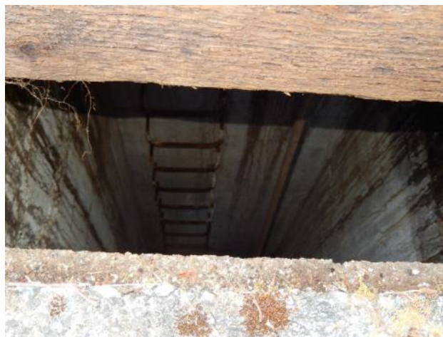
Figure 27: Reservoir drain valve chamber
