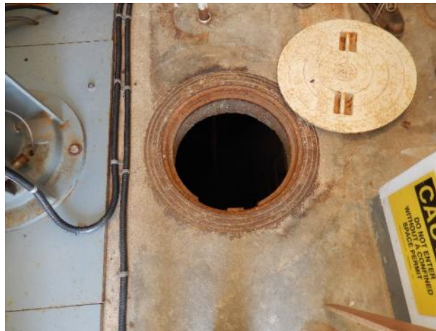
Figure 4: Stamp River pump house reservoir
