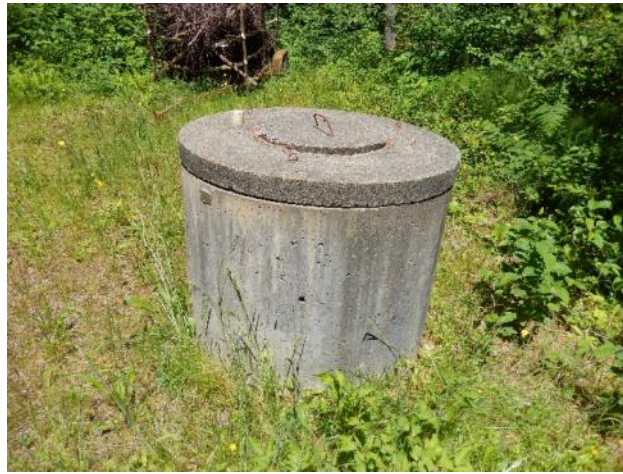
Figure 20: Main (#2) well head
