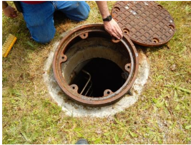
Figure 16: Karn Street pump house sump #1
