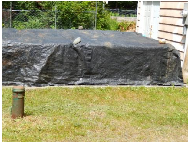
Figure 28: Manhole below salt storage area
