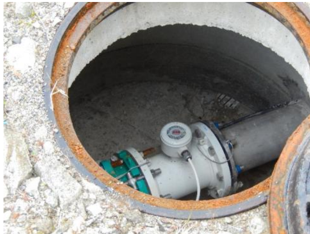
Figure 33: Meter chamber, reservoir compound
