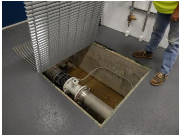
Figure 12: Strick Road pump station meter chamber
