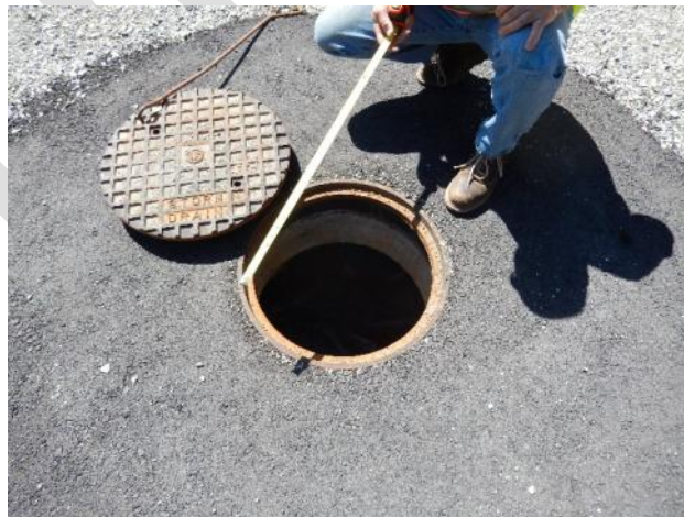
Figure 11: Kitsuksis drain line manhole
