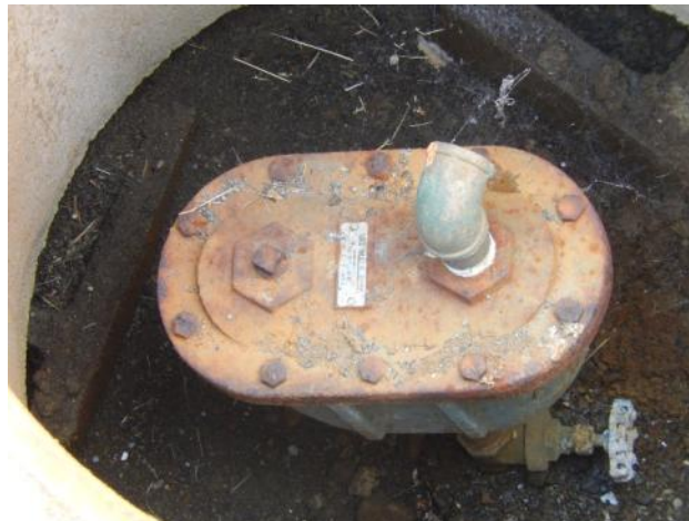
Figure 18: Karn Street air valve chamber
