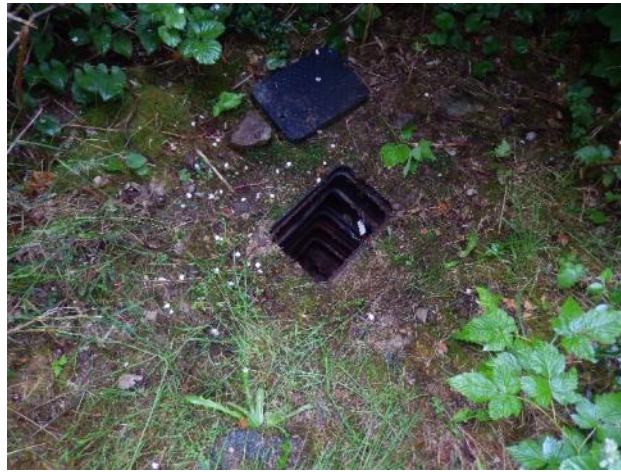
Figure 38: Parks Canada meter chamber
