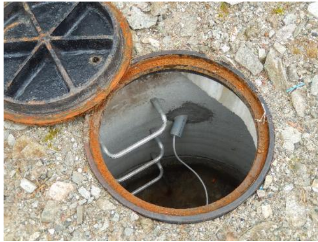
Figure 34: Rechlorination chamber, reservoir compound
