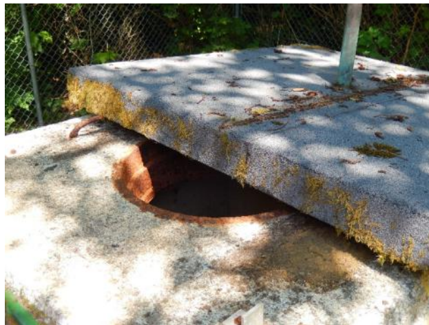
Figure 25: Reservoir inlet chamber
