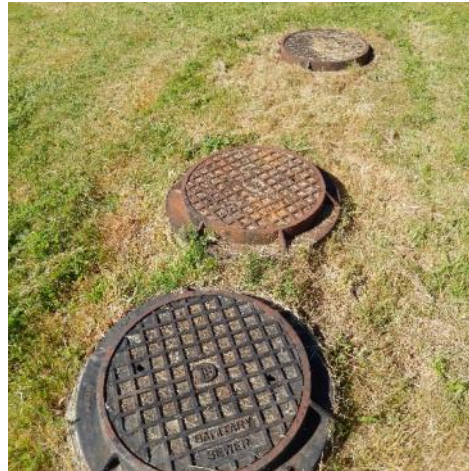
Figure 14: Office and maintenance building septic tank
