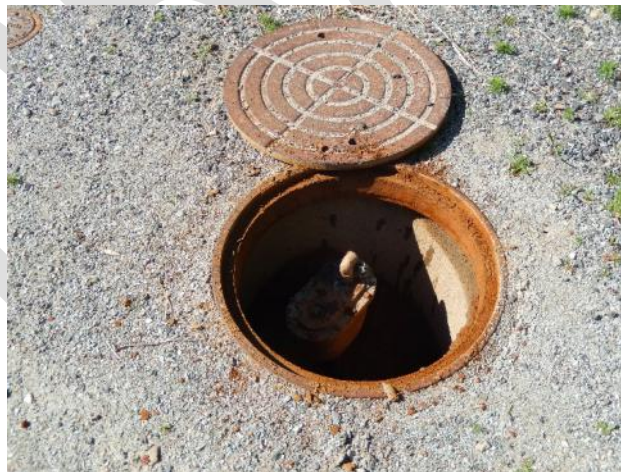
Figure 3: Beaver Creek north reservoir air valve chamber
