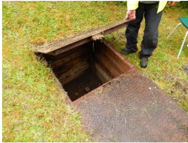
Figure 36: School meter chamber
