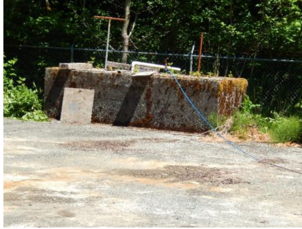
Figure 24: Reservoir valve chamber
