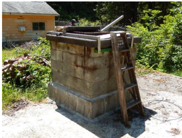
Figure 22: Reservoir main hatch
