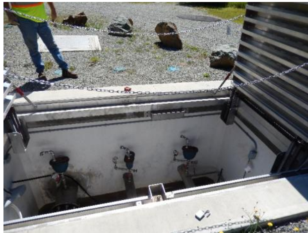
Figure 10: Kitsuksis air (altitude) valve chamber
