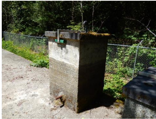
Figure 26: Reservoir old meter chamber
