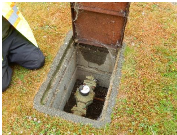
Figure 37: Hospital meter chamber
