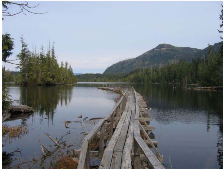
Photo 10. Bamfield Community Water System, Sugsaw Lake intake structure
