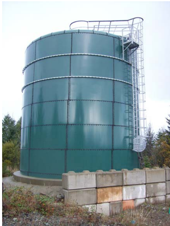
Photo 9. Alberni Valley Landfill Small Water System reservoir
