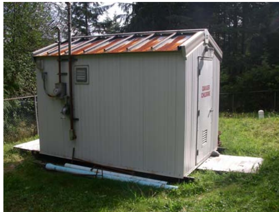
Photo 8. Millstream Community Water System pump house
