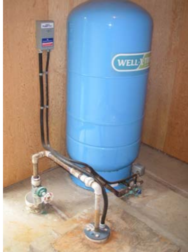
Photo 3. Alberni Valley Regional Airport pressure tank
