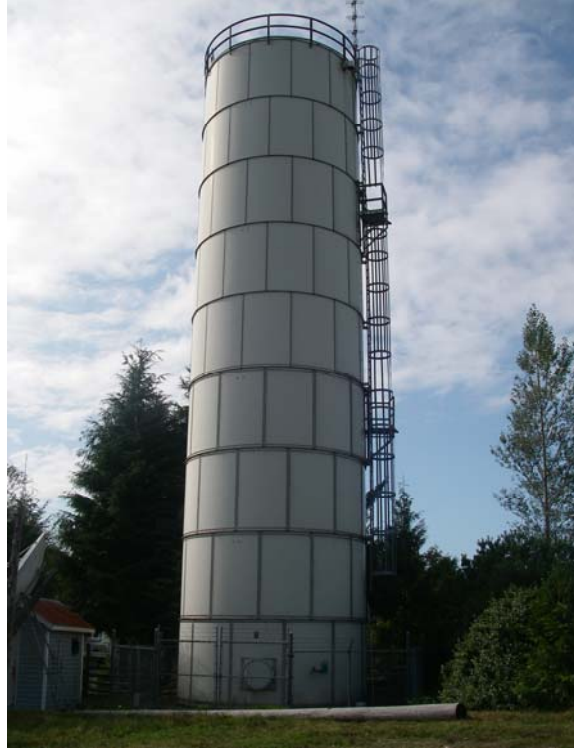
Photo 7. Millstream Community Water System reservoir
