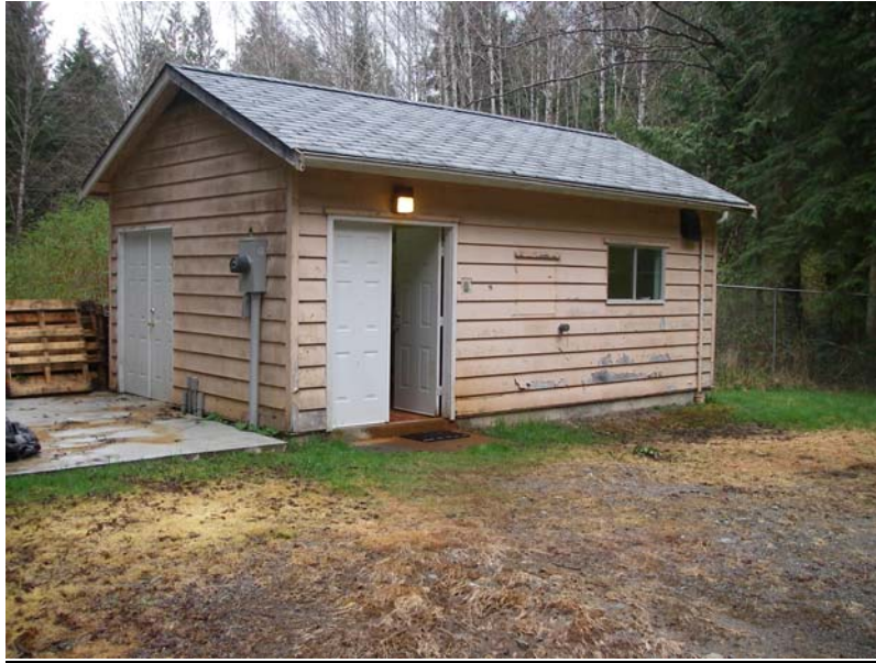
Photo 1. Tofino Airport Water System pump house
