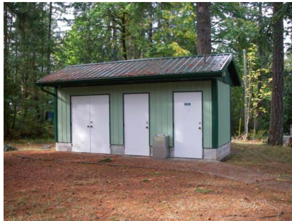
Photo 4. Cougar Smith Park water distribution and disinfection building
