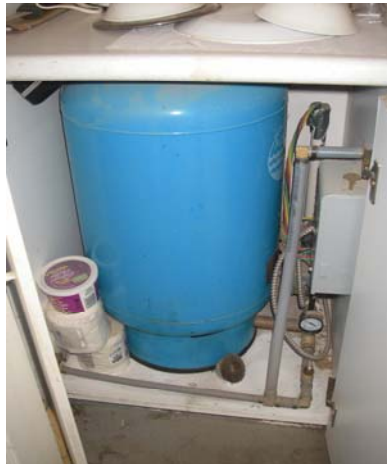
Photo 6. West Coast Landfill Small Water System
