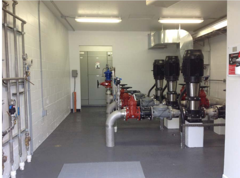
Strick Road Pump Station
