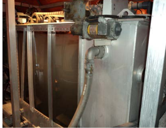
Dissolved Air Floatation Tank (DAF)
