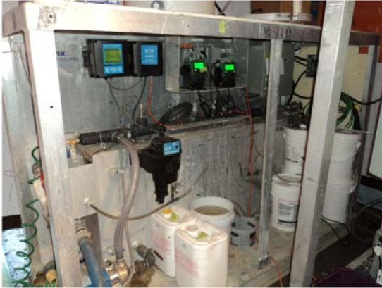
Raw Water Entering with Treatment Additives
