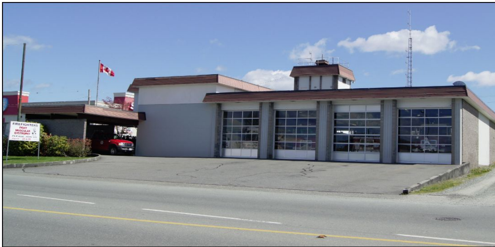
Figure 11: Port Alberni hall 1
