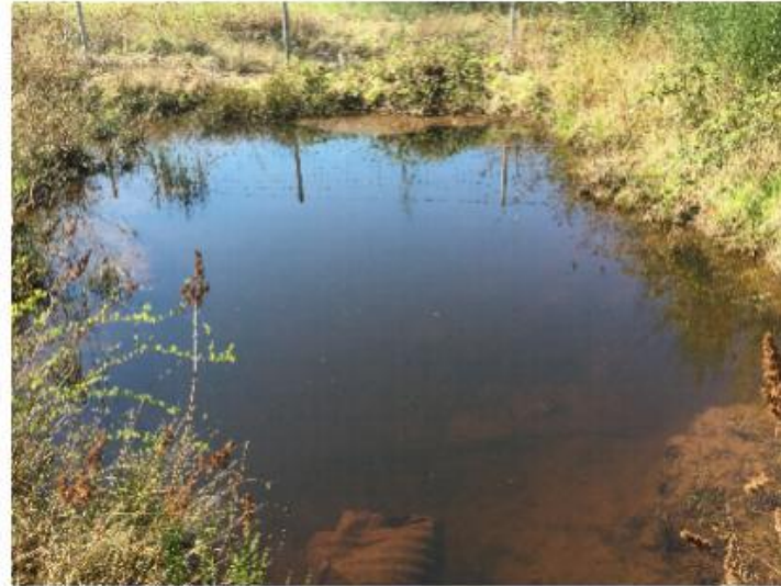
3.) Ditch 4 submerged culvert under service road.
