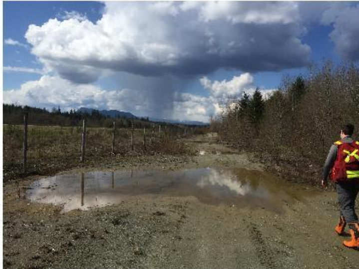
9.) Ditch 4/Beaver Pond overflow on road.
