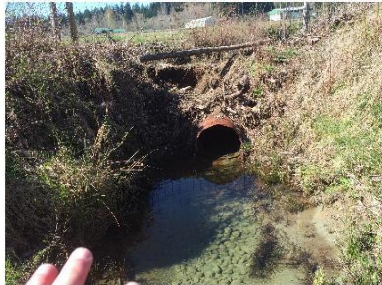
8.) Ditch 3 at runway culvert and end fish access.
