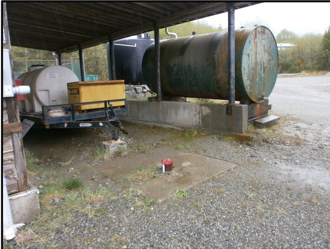
Well #10 – Looking North-West
