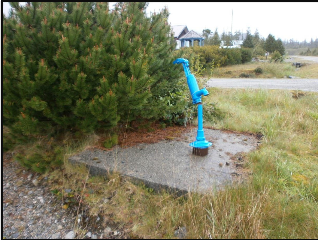
Well #12 – Looking North-West
