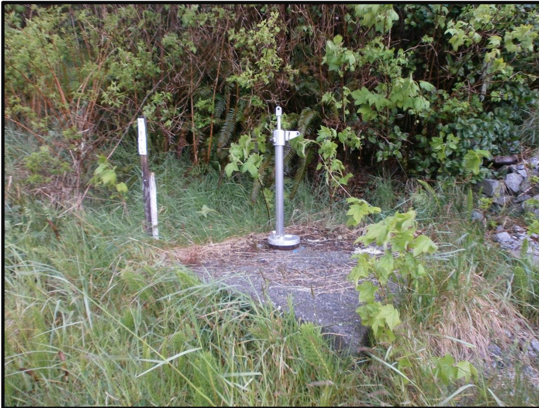
Well #19 – Looking North-West
