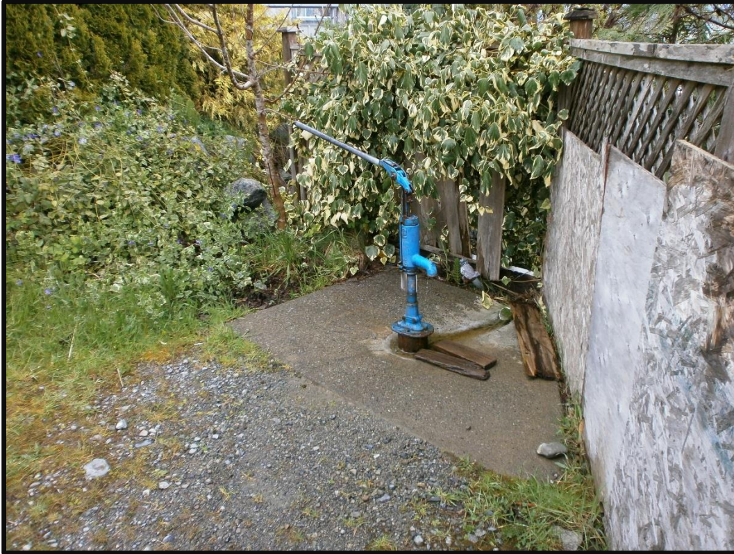
Well #17 – Looking North-East
